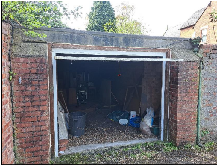
Photograph 1 showing the exterior of Building 1
