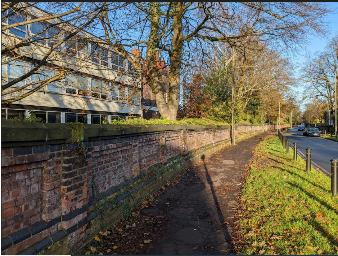
View north along Lower Park Road
