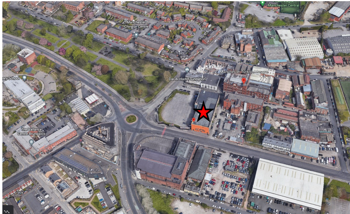
Aerial view of site with site marked with a star
