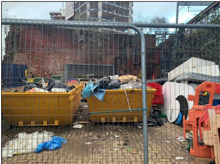
Photo 5 – Parcel 2 hardstanding with adjacent wall (W1)
