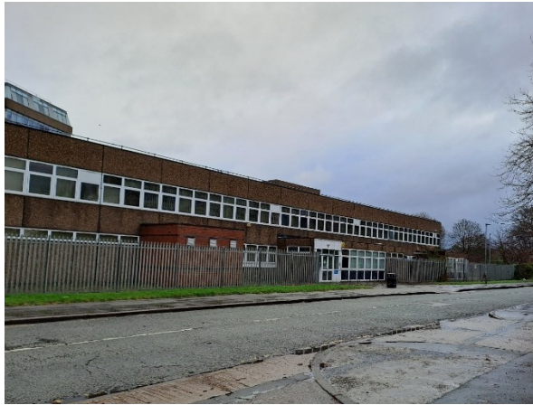
Views of Existing Building
