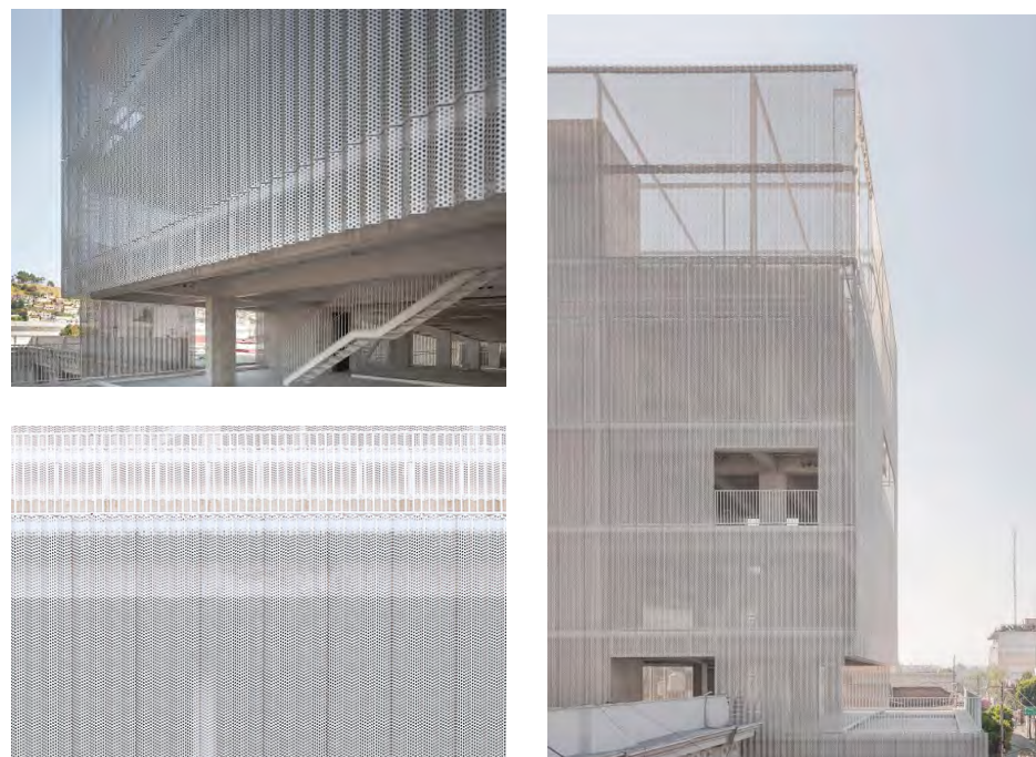
Fig 326 A veiled facade - FRPO, Estacion San Jose
