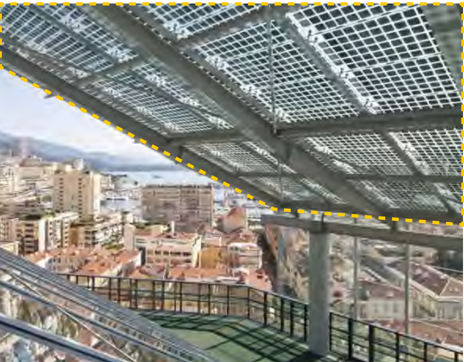
Fig 331 Precedent of a Roof canopy PV Application Ecole Hôtelière Monaco, France
