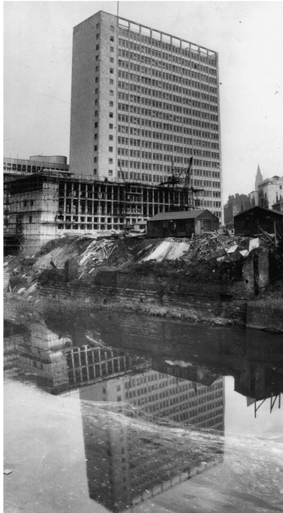
Fig 42 View East from the Salford side of the River Irwell with the low rise building along the Irwell still under construction. ca. 1959
