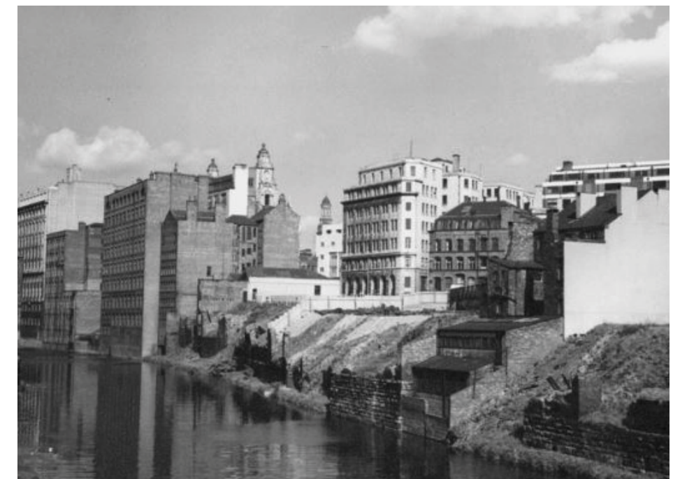
Fig 34 Albert Bridge House on the right of the river prior to construction with site hoarding (1957)
