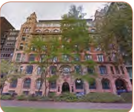
Image of Listed Building 6: Century Buildings Grade II. 06/06/1994
