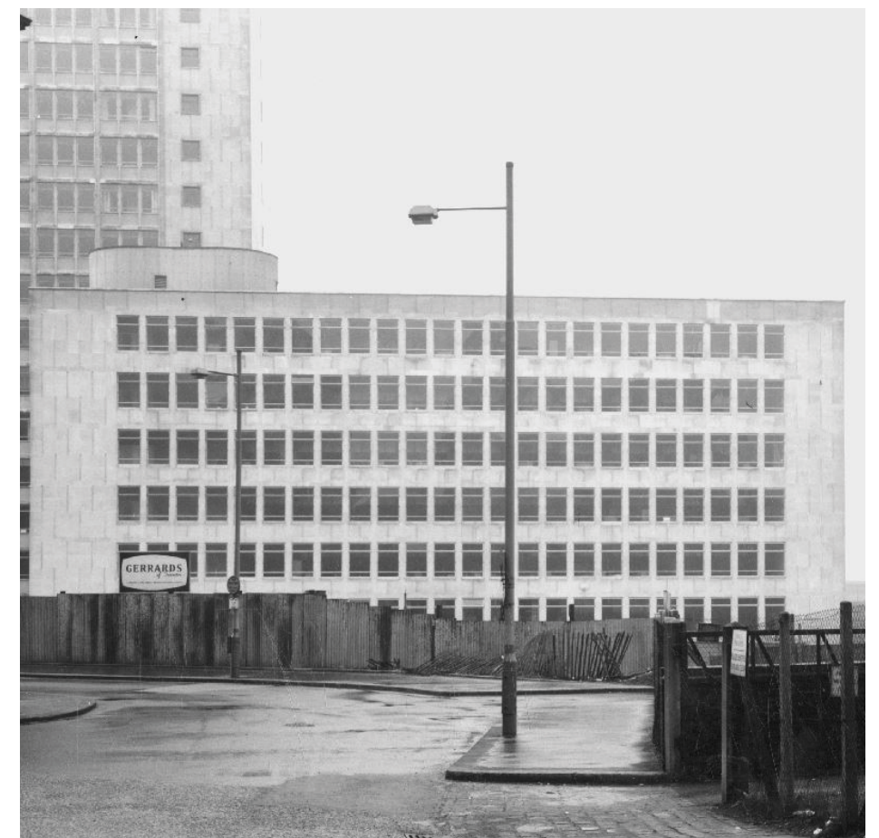
Fig 43 View west along St. Mary's Parsonage with the Albert Bridge House development recently constructed (1959)
