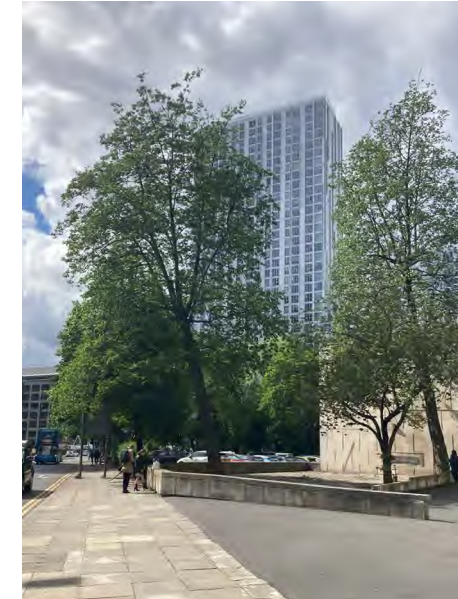
Fig 60 Trees subject to TPO
