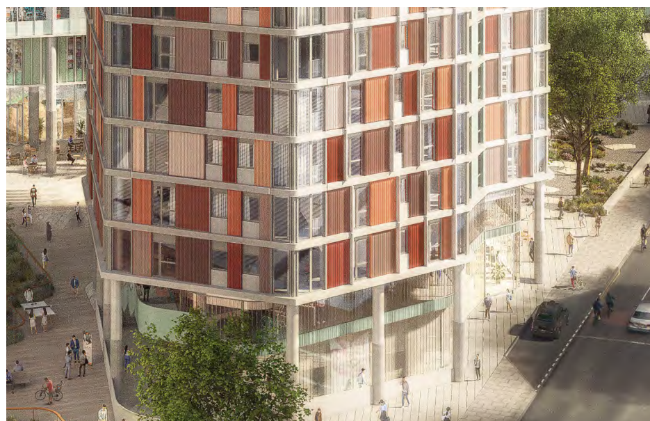
Fig 237 Materiality - Aluminium corrugated panels in varying rust tones
