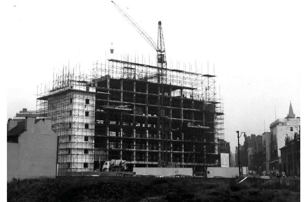
Fig 41 Construction of Albert Bridge House underway facing East (1958)
