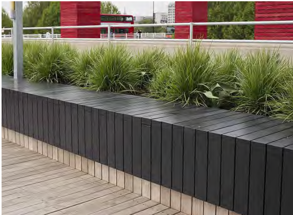
Fig 177 Decking material being used to form a linear seating element
