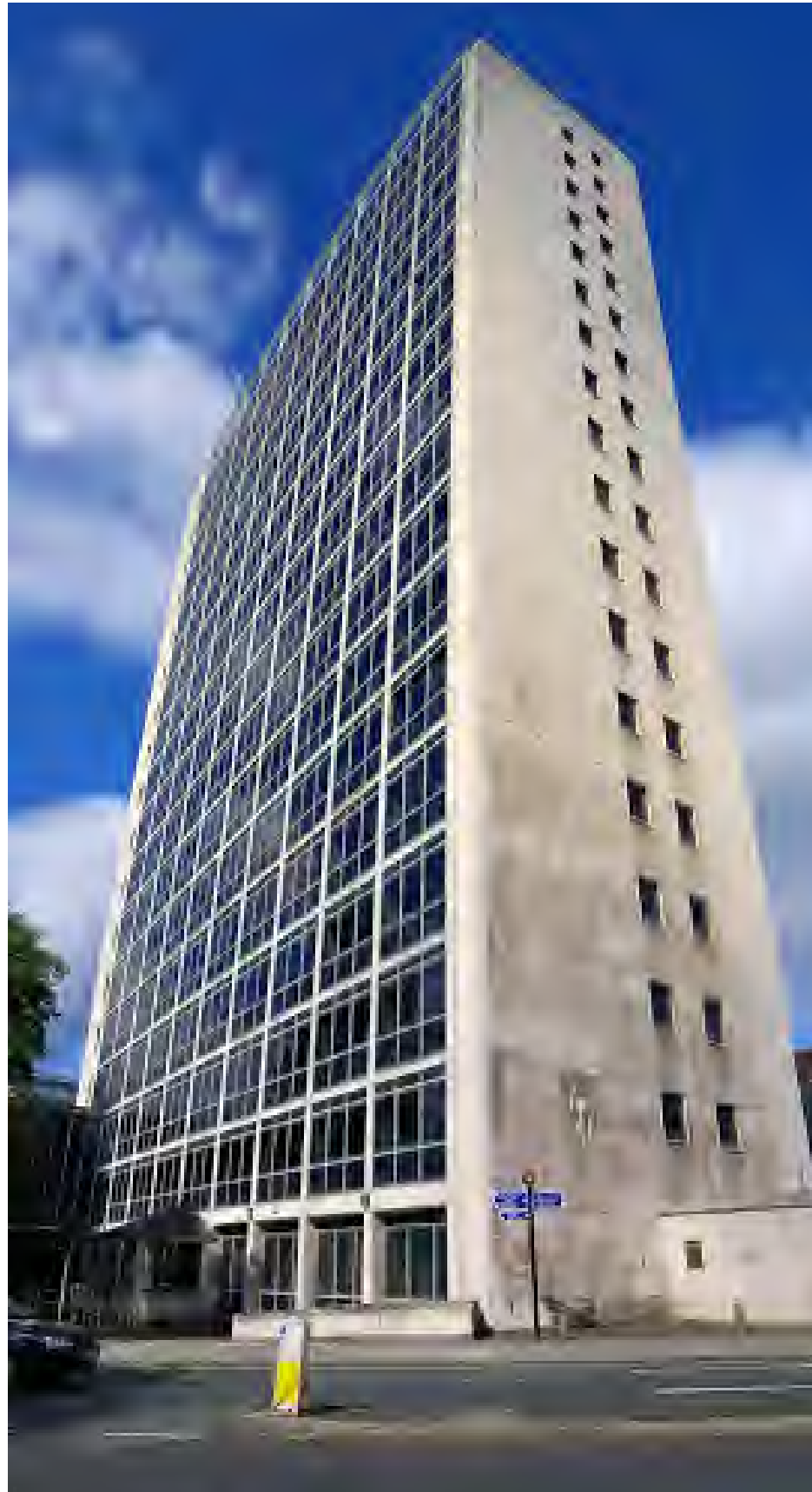
Fig 44 Alberton Bridge House (2022)
