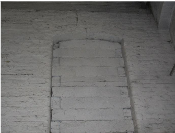
Photo 27: No bats or suitable gaps for bat access found around the blocked up doorway apertures
