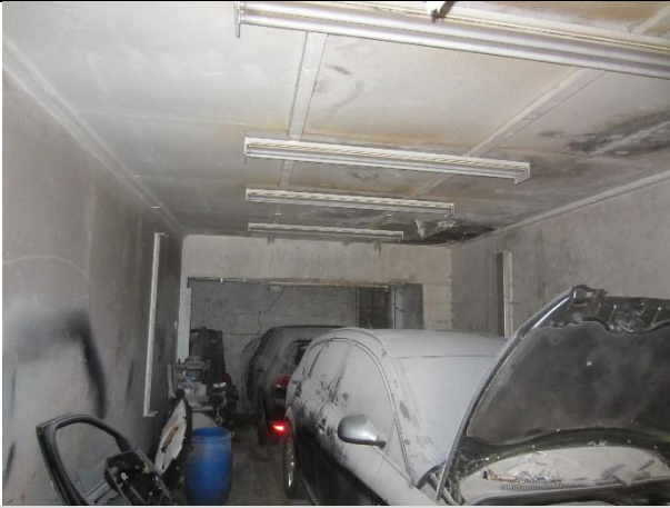
Photo 19: Interior of B3
