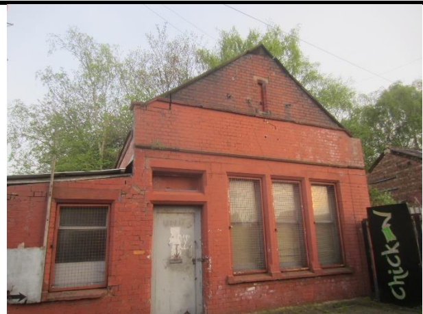
Photo 8: Norther elevation of B2
