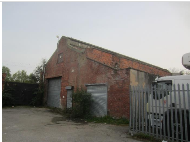
Photo 22: Eastern elevation of B4
