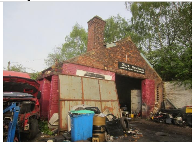
Photo 12: Western elevation of B3
