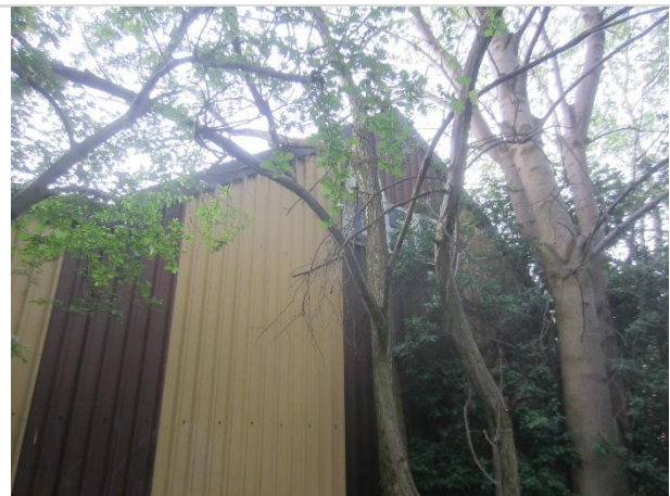
Photo 10: Southern elevation of B2 showing metal cladding and tree / shrub cover
