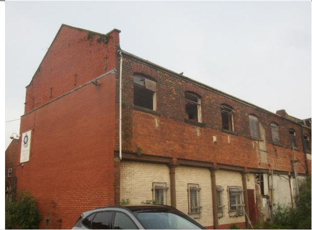
Photo 2: Northern and western elevations of B1
