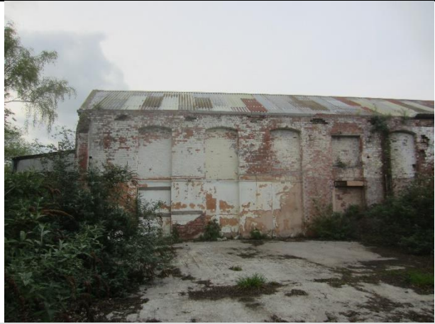
Photo 20: Southern elevation and roof of B4
