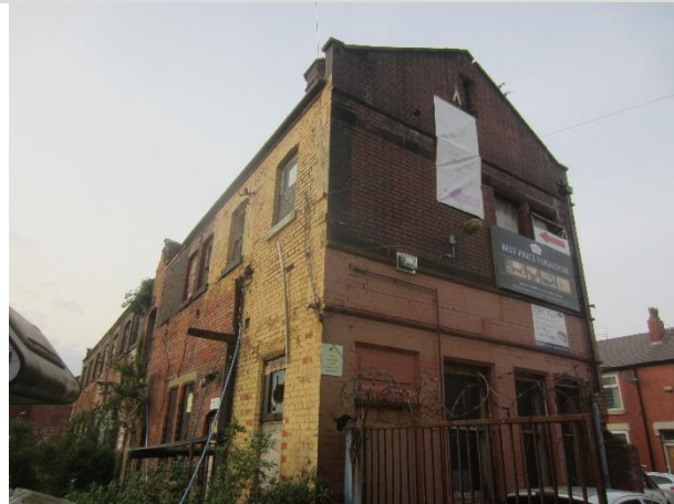
Photo 5: Western and southern elevations of B1
