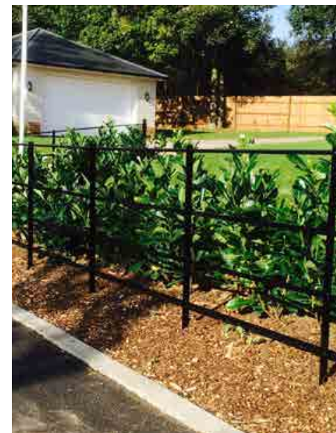
BOUNDARY TREATMENTS - PARKLAND FENCING
