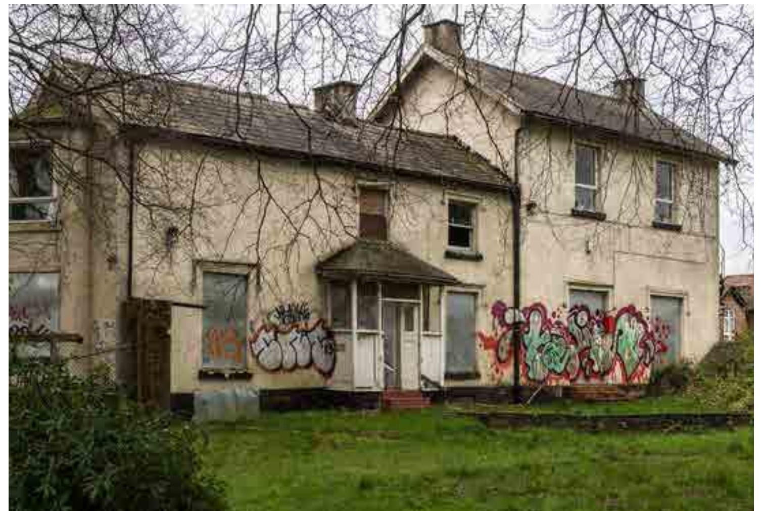
Nello James Community Centre - Present Day
