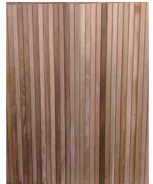
BOUNDARY TREATMENTS - 2M VERTICAL CEDAR FENCING TO MATCH TIMBER ELEMENTS ON HOUSES
