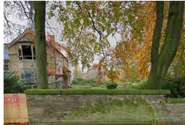
Overgrown land to north of building
