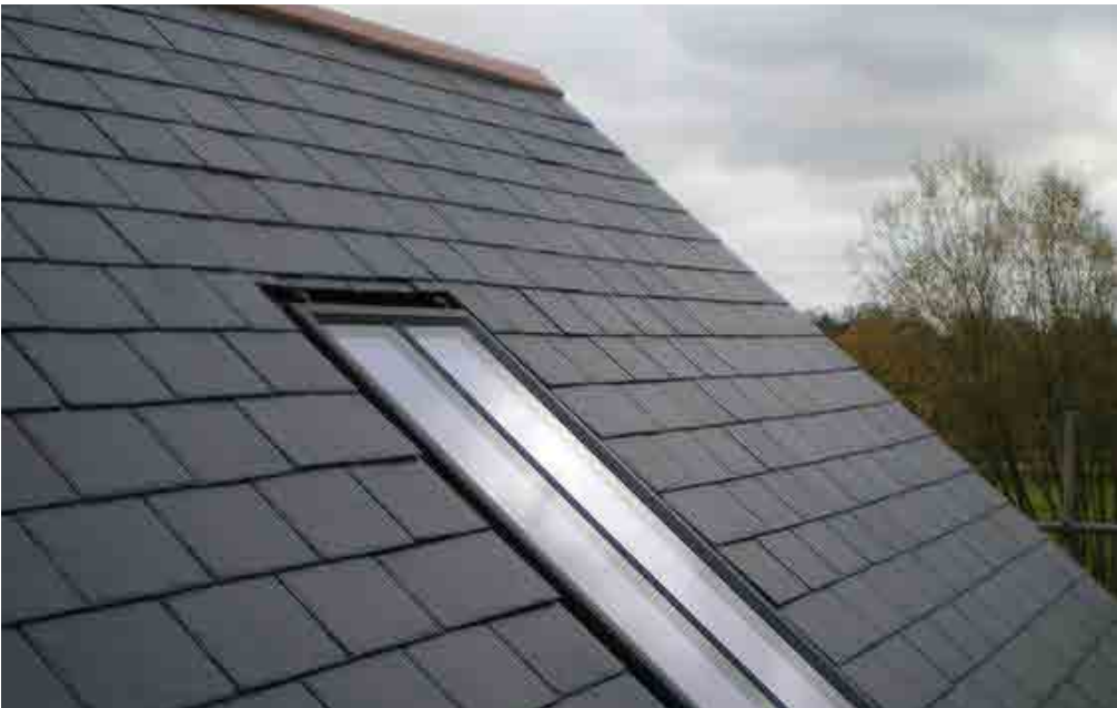
CONSERVATION ROOFLIGHT FLUSH IN GREY TILED ROOF
