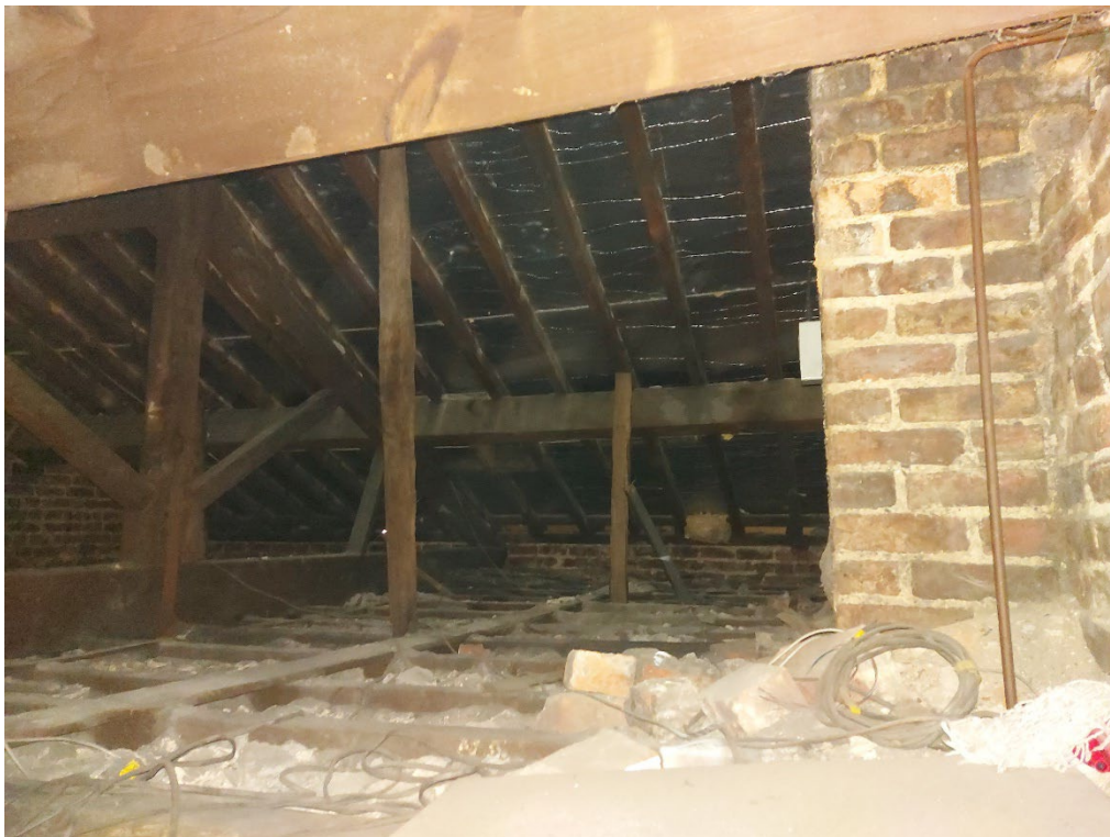
Photograph 4 Opposite elevation appears to be in good condition. Reflective silver felt over (difficult to discern on photograph), obviously recent
