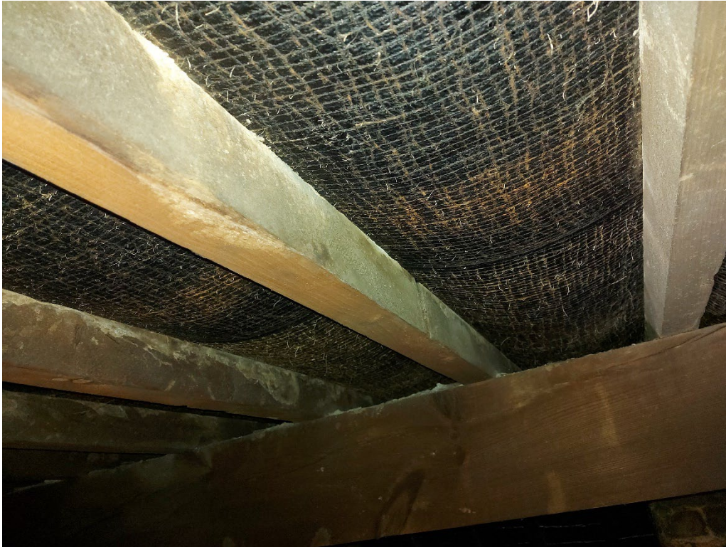
Photograph 3 Oxford Road side – roofing felt in good condition
