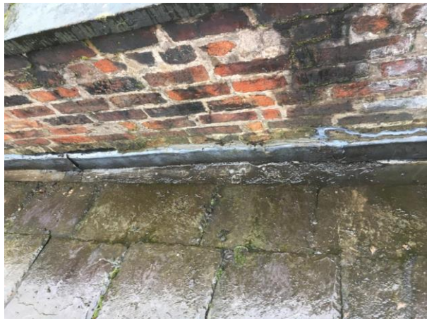
Lead reinstated and mastic applied.
