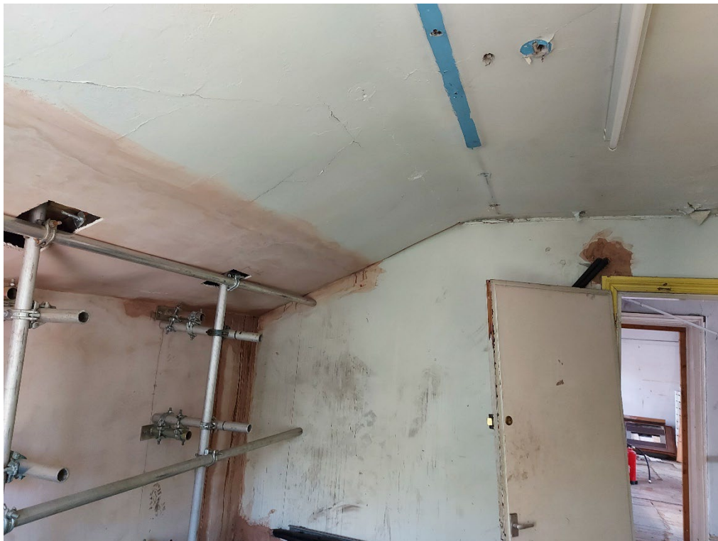
Photograph 6 Rear annexe (Dover Street side) – scaffold support to parapet wall over
