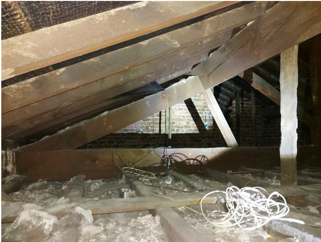
Photograph 1 View of roof from access hatch – traditional cut rafters and purlins, king post truss at mid-point
