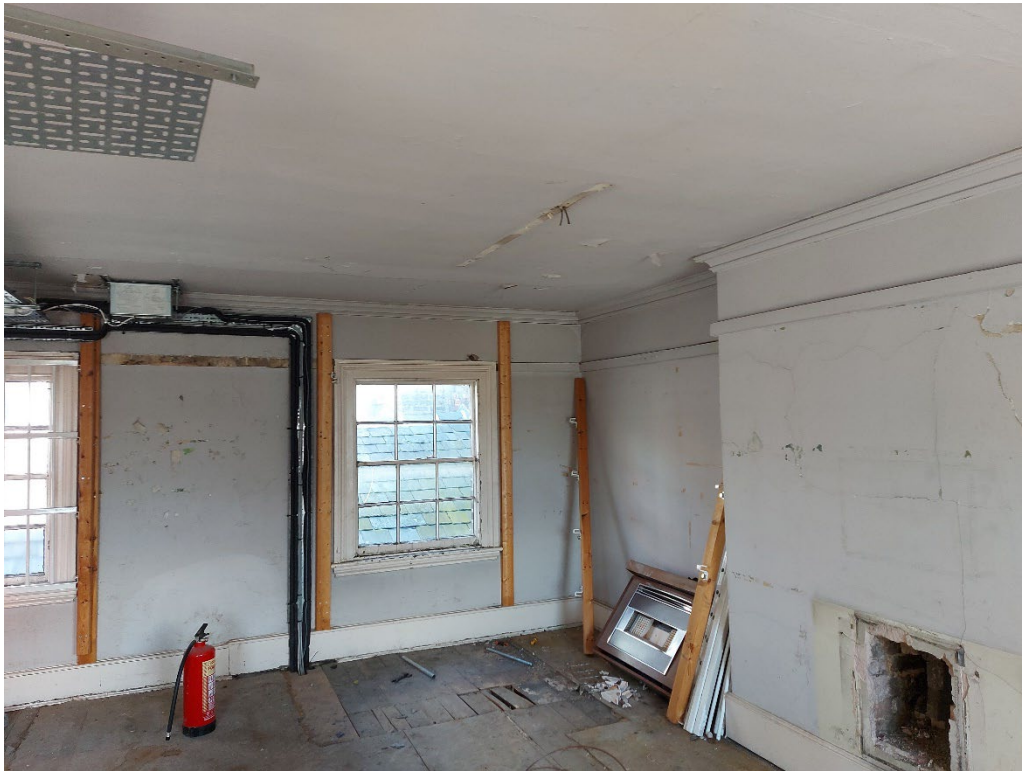
Photograph 5 Ceiling soffit generally in good condition, no cracking
