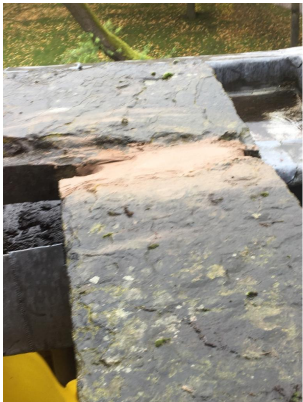
Coping stone joint re-pointed.
