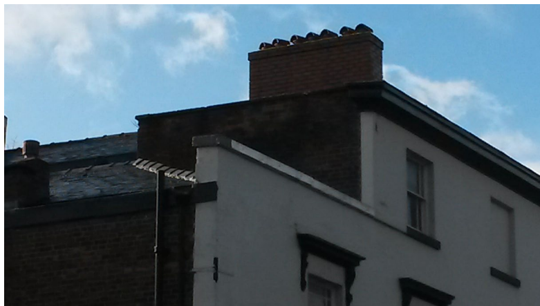
Rear view of existing parapet, from Dover Street
