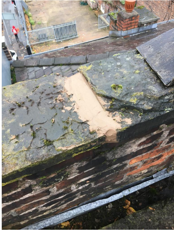
Coping stone joint re-pointed.
