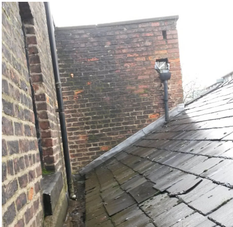
Photograph 8 Parapet wall (from rear window)
