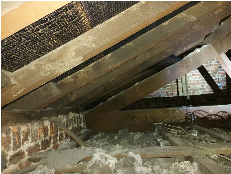
Photograph 2 View on eaves (Oxford Road side) – timbers appear to be in good condition. Substantial ceiling joists
