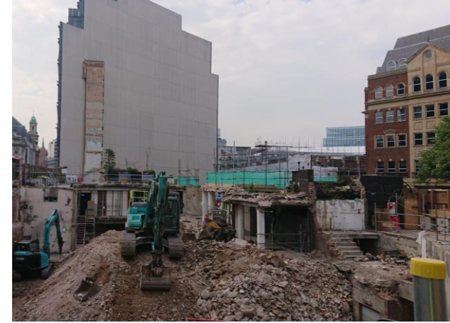
Works on site at Holborn
