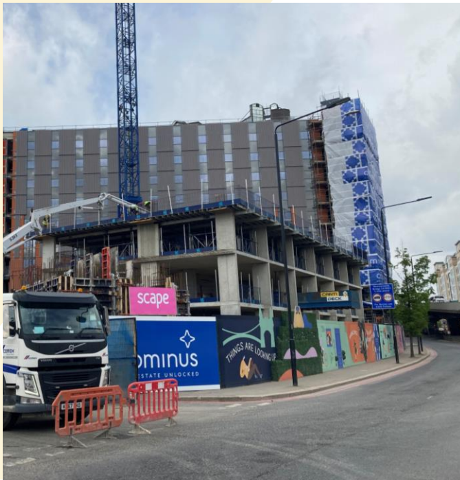
Works on site at Hammersmith
