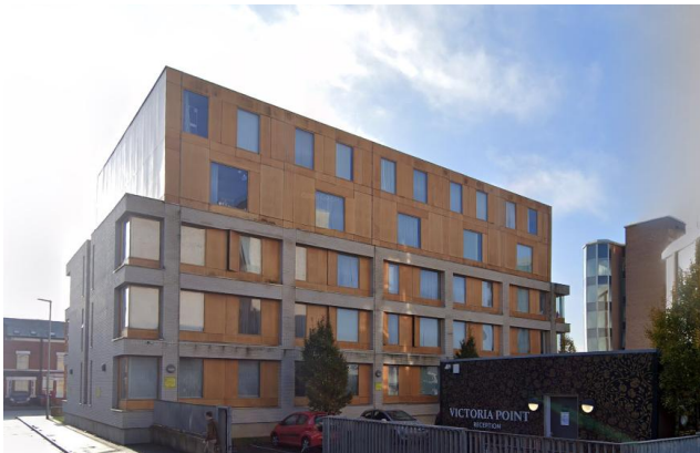
Victoria Point, Bay Road
