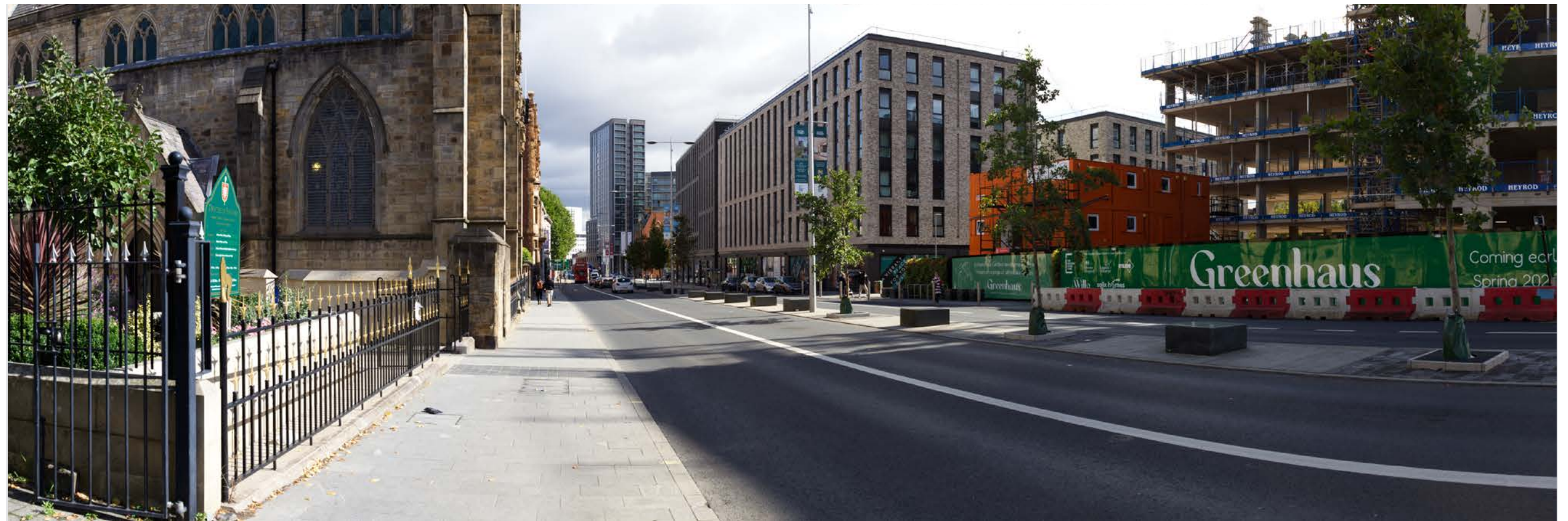
Verified View - Viewpoint 30 Junction of Chapel Street and Great George's Street - Existing - RAD
