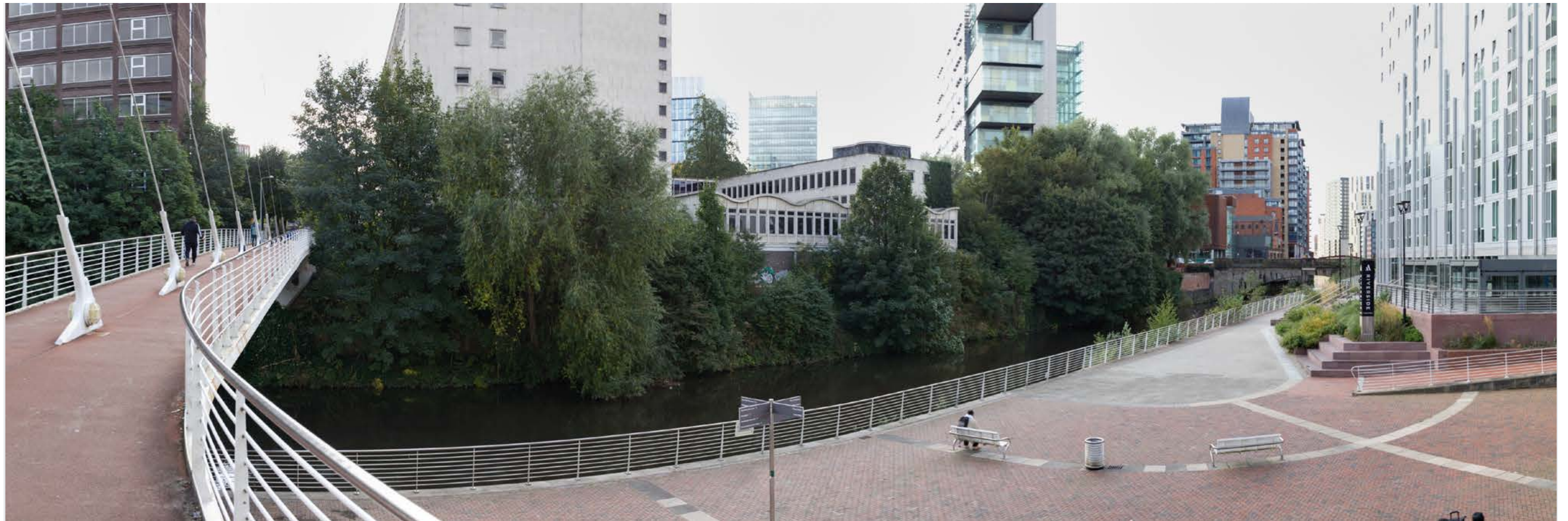
Verified View - Viewpoint 1 Trinity Bridge adjacent to Clermont - Ferrand Square - Existing - RAD
