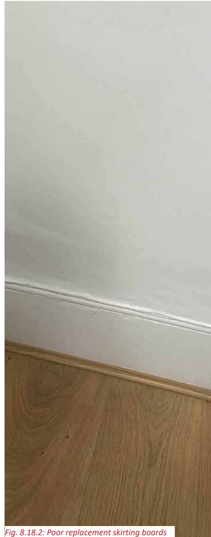
Fig. 8.18.3: Poor replacement skirting boards
