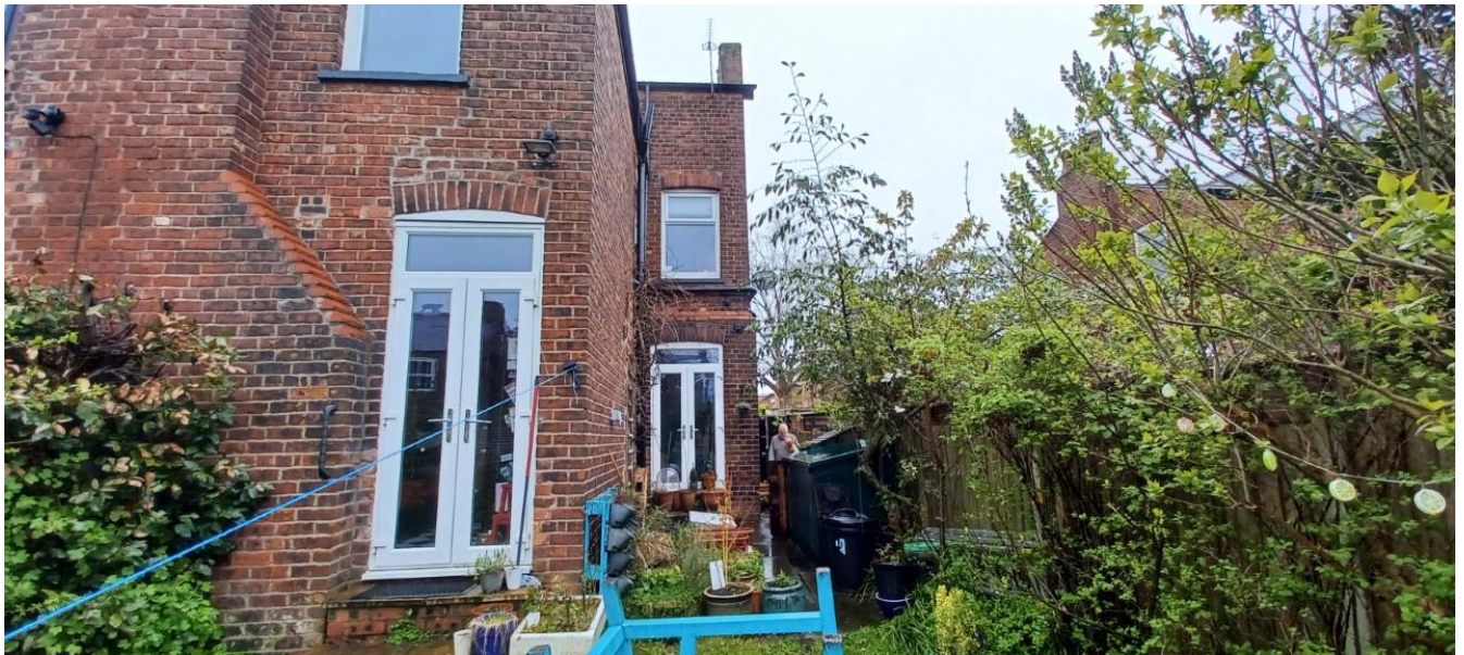
Figure 2. Rear view of property.
