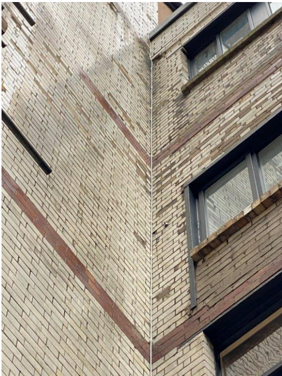
Image 3.3: Conductor Tape – Courtyard
