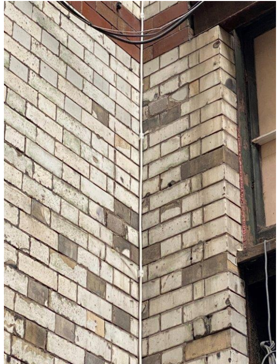
Image 3.2: Conductor Tape – Courtyard
