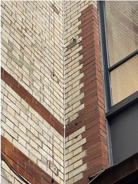
Image 3.1: Conductor Tape – Courtyard
