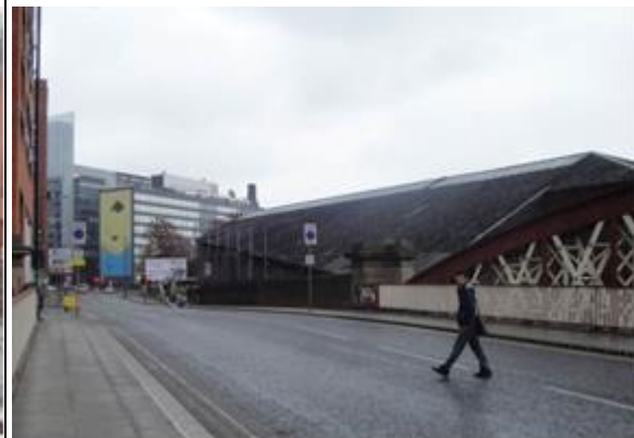
Figure 21: View of Albert Shed (east side) from Irwell Street Bridge. Note the slanted, asbestos tile roof
