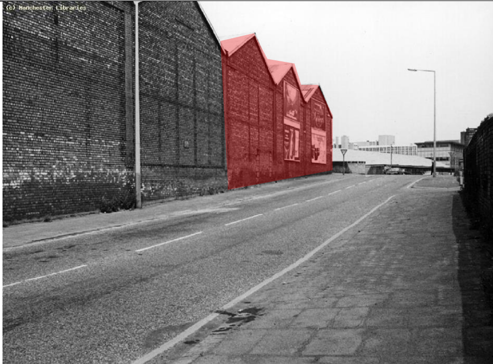
Figure 17: Historic Image (1973) Water Street , looking east pictured c.1973. Illustrates the 5-bays to Albert Shed (three shaded red are all that survive). The distinct stone to the third bay within the image denotes the location to the former wing to Albert Warehouse is pictured prior to having been developed into a hotel in c.1980s. The southern shed (now demolished) is glimpsed to the left side of the image.
