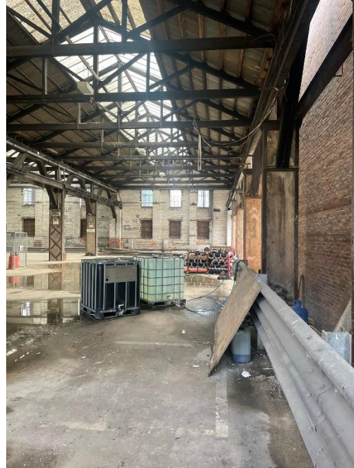
Figure 27: Looking south along western shed. Note the external wall to 1990s extension.
