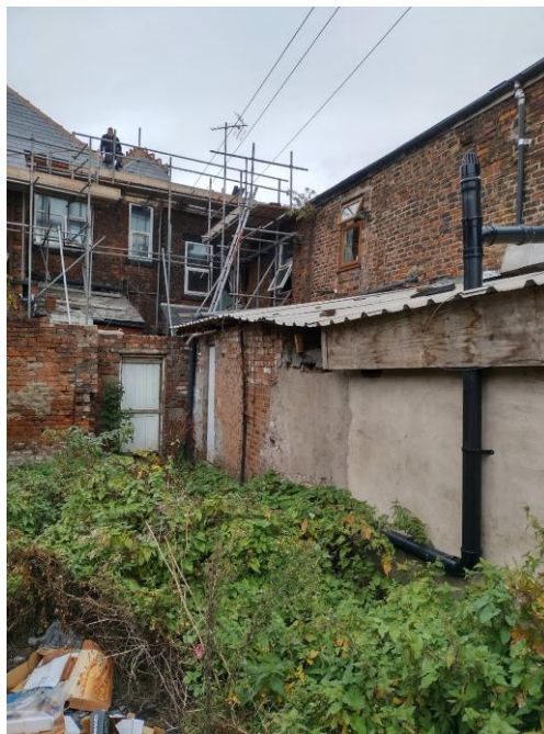
Fig.2 – Rear of 940 Stockport Road
