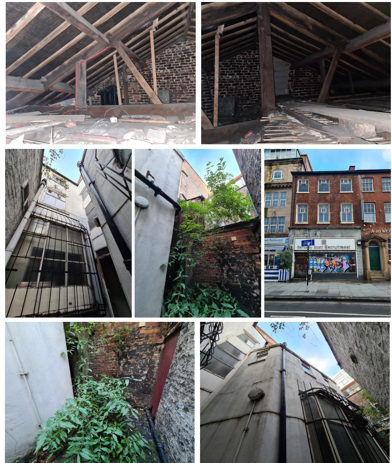
Figure 6: Top – Roof Void, Middle – Rear + Front Elevations, Bottom – Rear Elevations
