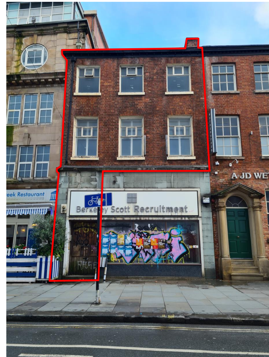
Figure 1: Front elevation of 65 Princess Street
