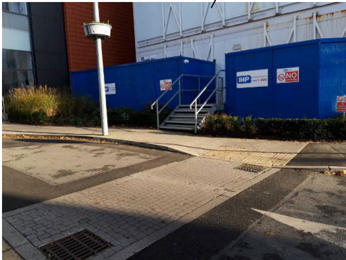
View to the east - IHP site cabins
