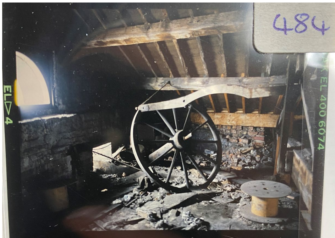
Figure 9: GMAU photographic archive contact sheet ref: 48 4.484. Bay 2 close to one of the lunette windows showing sarking boards over the common rafters, an alternate finish beneath the slates.
