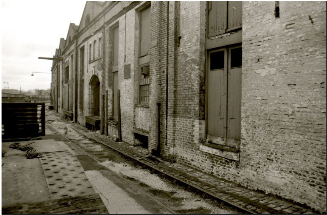
Figure 6: n.d photograph of the eastern part of the southern elevation (Manchester libraries, supplied by museum)
