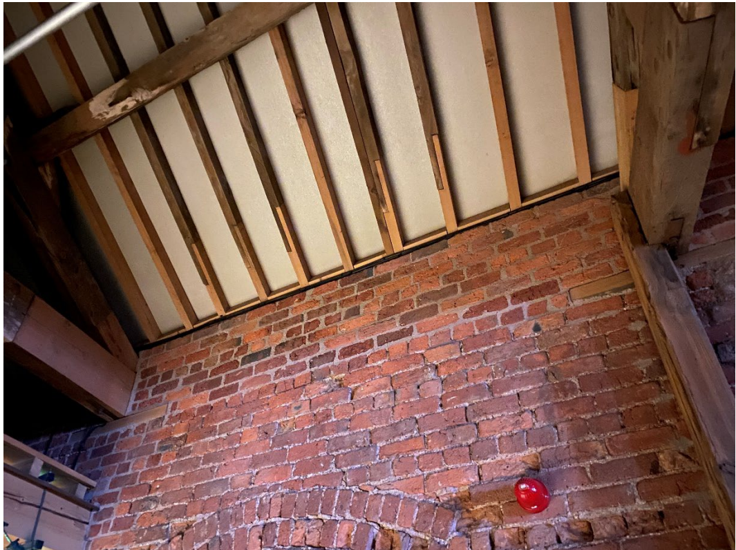
Figure 15: View towards one of the party walls between the bays showing scarfed in timber replacements to the common rafters and a change in the brickwork between the trusses suggestive of rebuilding to enclose the valley gutters.
