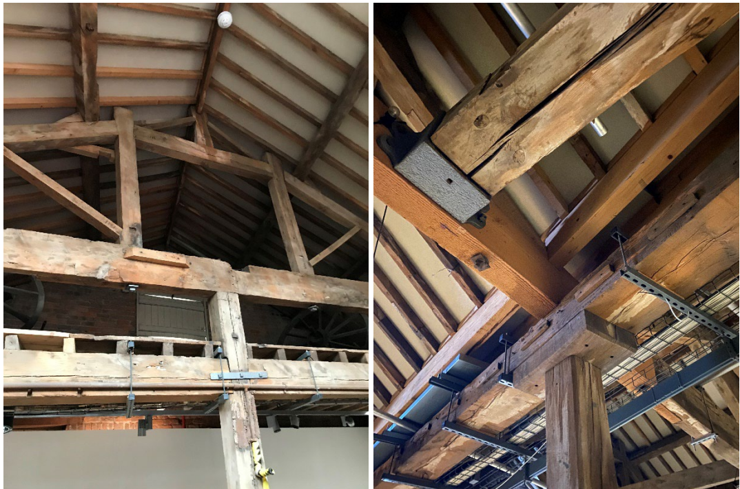
Figure 13-14: (left) one of the principle roof trusses (Bay 2). (right) valley gutter in Bay 2 showing modern purlins beneath the gutter and above the historic beam, drip tray visible bottom left.
