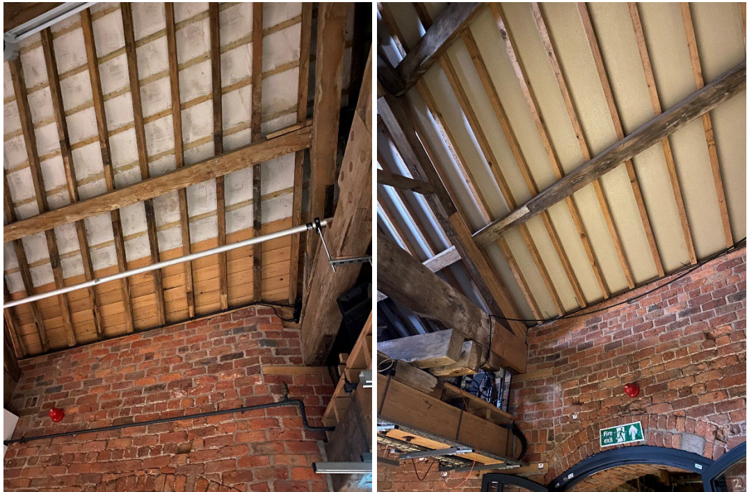
Figure 11-12: Bay 4 on the left with sarking boards reflecting the position of the valley gutter and the visible battens with torching and (right) Bay 3 with continuous boarded finish above the common rafters.
