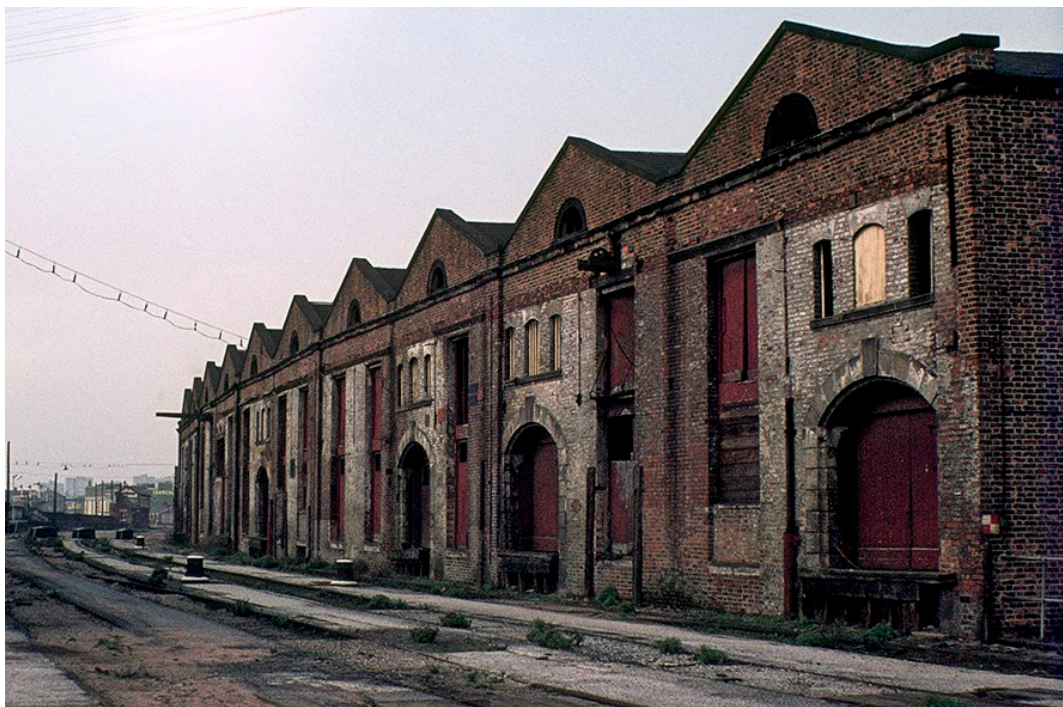
Figure 5: n.d image of the southern elevation from Bay 5 looking west prior to works. (Manchester Libraries, supplied by museum)
