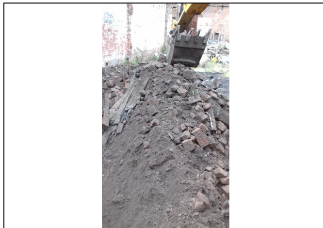
Trial Trench 103A Spoil
