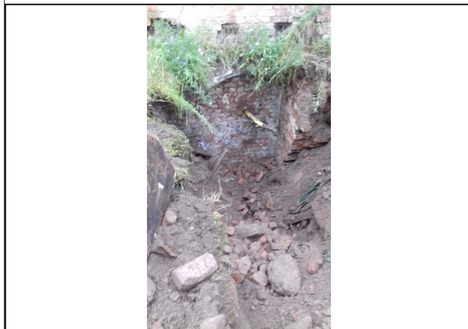
Trial Trench 103A
