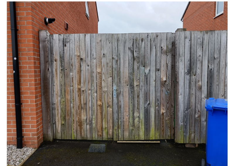
Photo - Existing Gates and Fence
