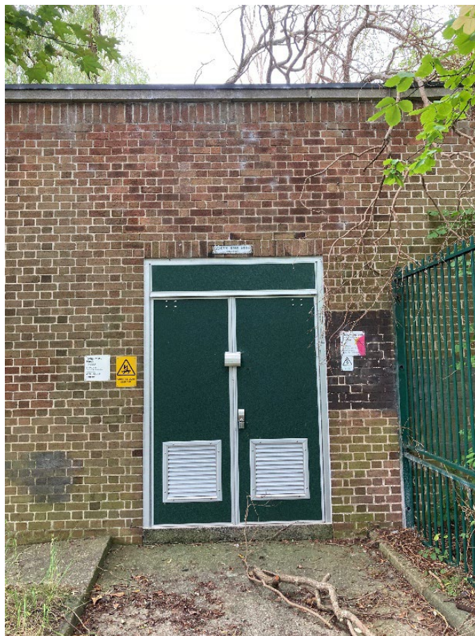
Photographs 1 - Building housing electric mains.
