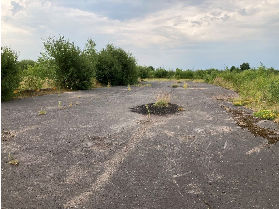
Photograph 8 - Areas of hardstanding in the west and south of Site
