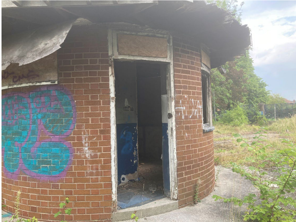
Photograph 3 - Security hut near entrance.
