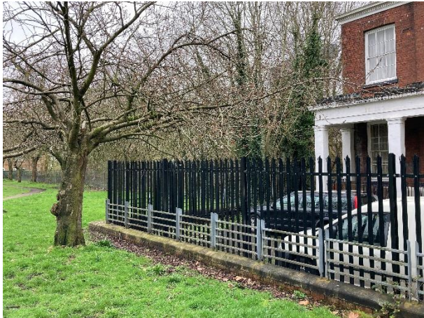
3.19: View of the front of Hulme Barracks and adjacent land that is closed off from public access.
