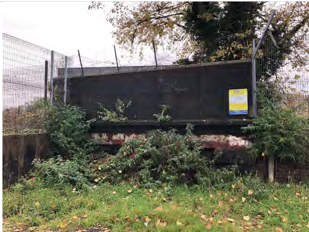
PLATE 6 EVIDENCE OF FORMER CANAL BRIDGE.
