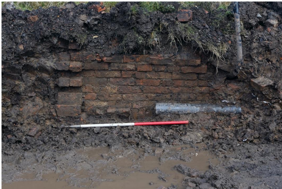
Plate 2 Wall [1012] & truncating sewer pipe
