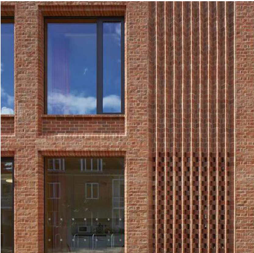
Vertical Brickwork Detailing
