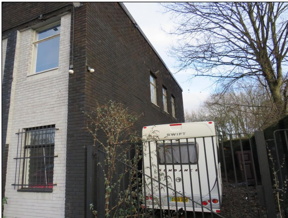
Photograph 4; A view of the south end of the building, the roof and wall joints are sealed by fabricated facias.
