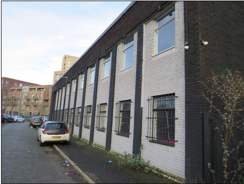
Photograph 3; A view of the western face of the building, note the condition, no gaps or crawl space were noted during the survey.
