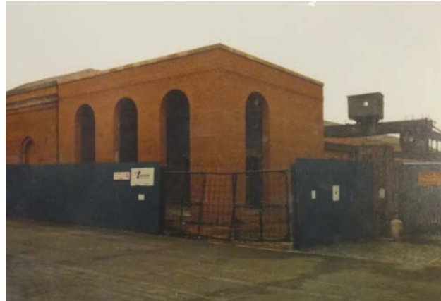
2.22 c.1983 View of the Visitor Entrance Block (SIM Archive YA2007.4129. Licence CC-BY-NC-SA 4.0)
