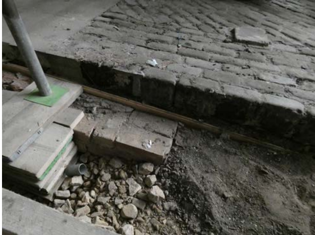
A.35 Cobbles with modern brick underneath (Insall).
