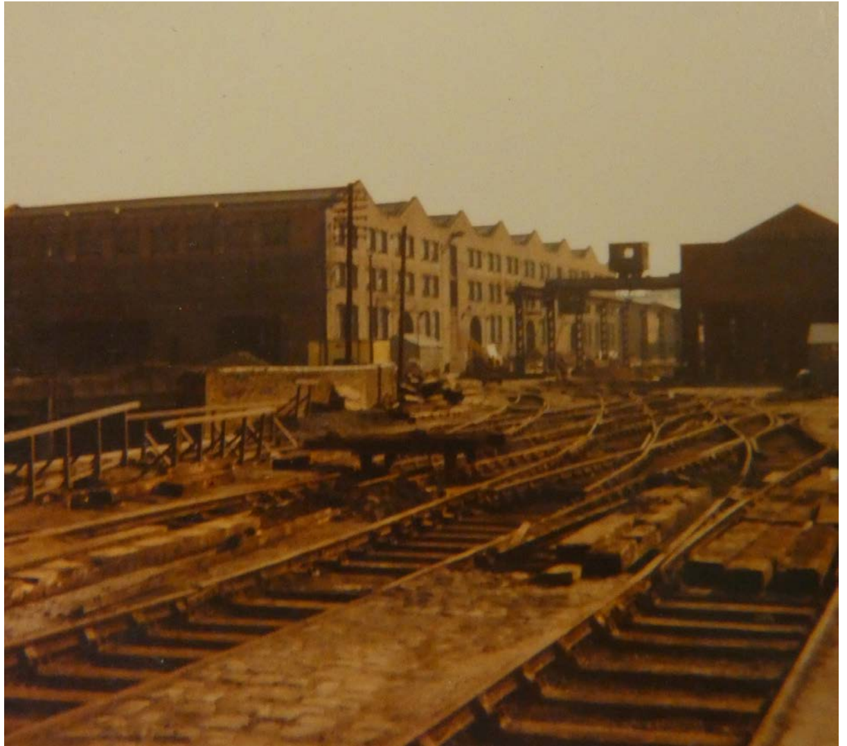
2.12 View of Upper Yard to Power Hall (SIM Archive YA2007.4129. Licence CC-BY-NC-SA 4.0)
