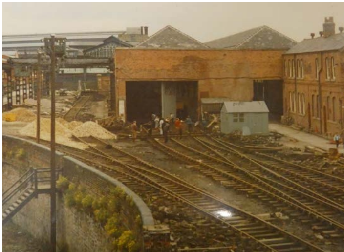
2.13 c.1980 Photograph of the Power Hall and Upper Yard (SIM Archive YA2007.4129. Licence CC-BY-NC-SA 4.0)
