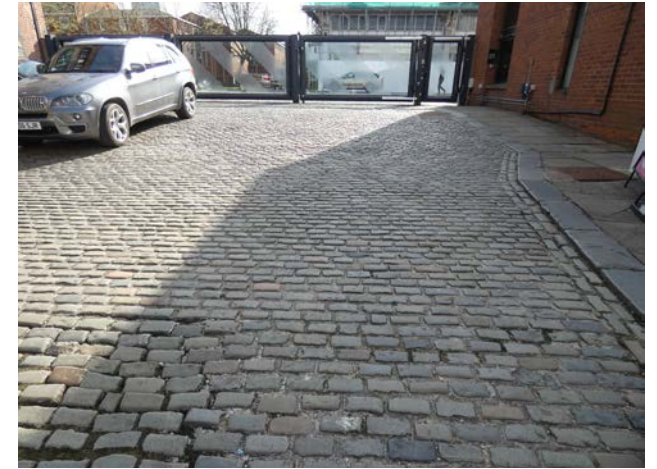
A.5 Setts in the Upper Yard, close to the entrance (Insal).
