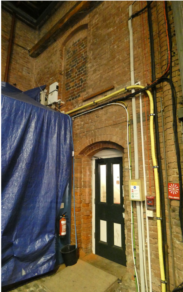
A.19 Doorway to the former Goods Offices (Insall).
