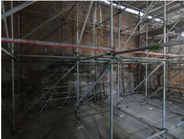
A.24 View of the east wall (Insall).
