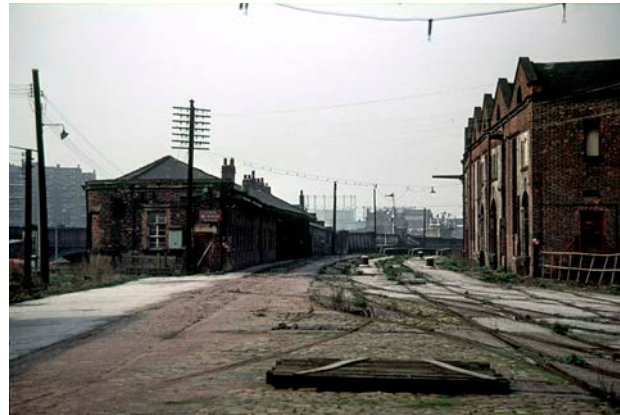
2.6 1830 Station and Warehouse in 1975 (MMU Visual Resources Centre)
