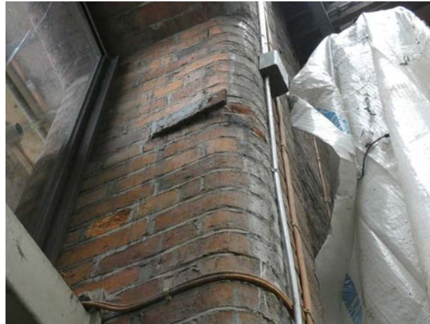
A.22 Metal plates within carriage door reveals (Insall).
