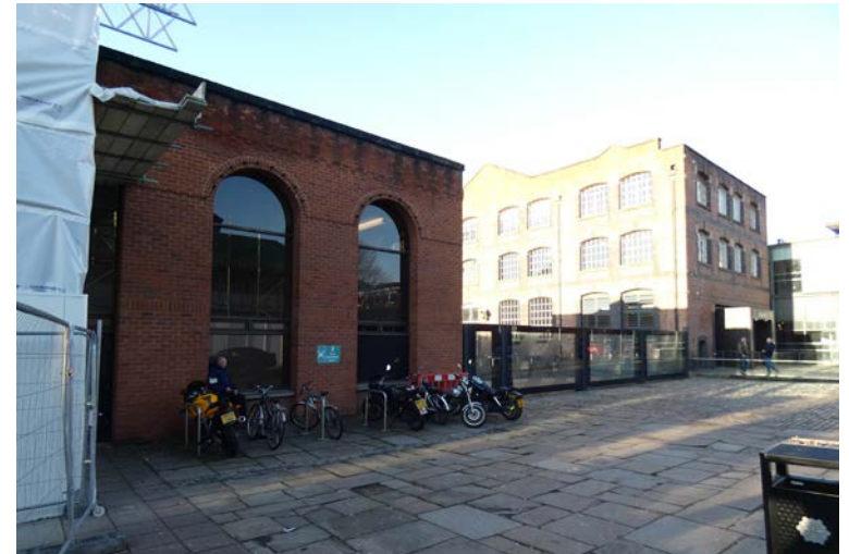
A.14 East elevation of the 1980s extension (Insall).
