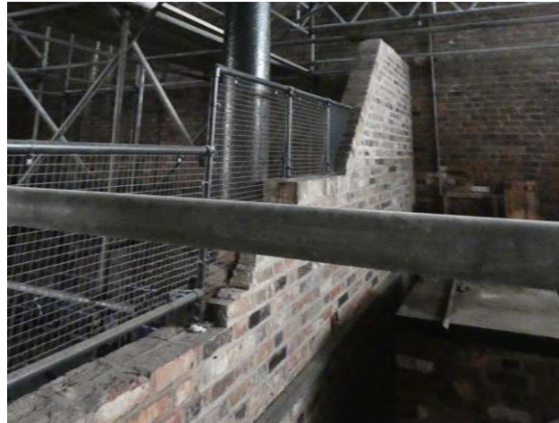
A.25 Modern brick abutment (Insall).
