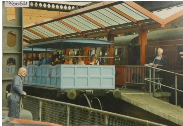
2.24 1980s platform in the Upper Yard (SIM Archive YA 2007.41)
