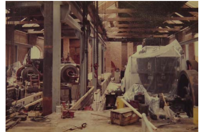
2.20 c.1983 View of the Power Hall (SIM Archive YA2007.4129. Licence CC-BY-NC-SA 4.0)
