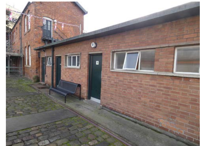
A.8 Toilet Block west of the Power Hall (Insall).
