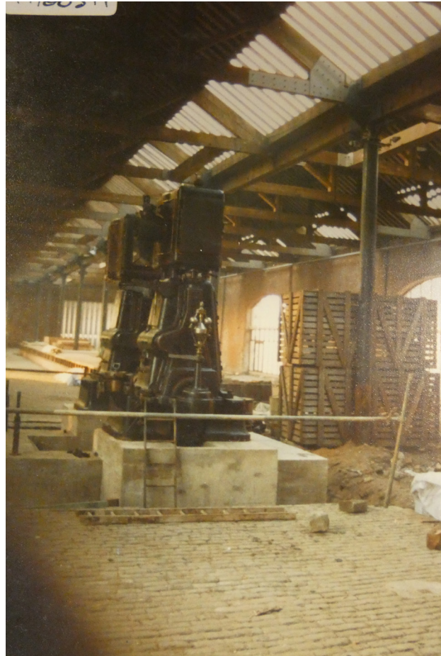
2.18 c.1981 View of the Power Hall (SIM Archive YA2007.4129. Licence CC-BY-NC-SA 4.0)
