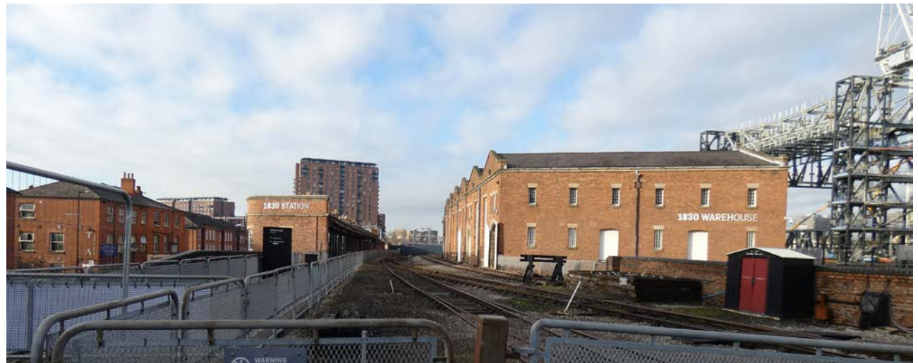
A.3 1830s railway buildings, west of the Power Hall (Insall).
