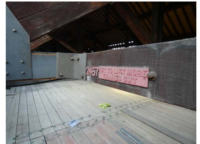
A.31 Interstitial beam for crane (Insall).
