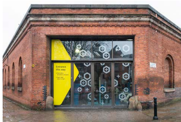
A.1 The splayed corner of the Power Hall (SIM).
