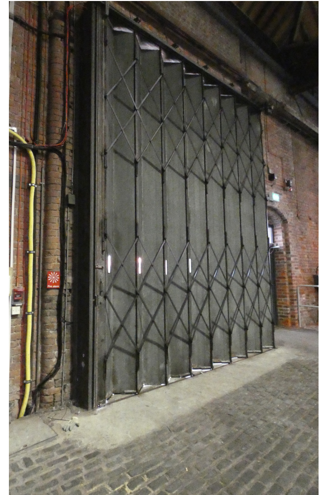
A.18 Former roadway entrance in the west wall (Insal).
