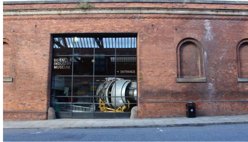
A.10 The western opening on the south elevation (SIM).
