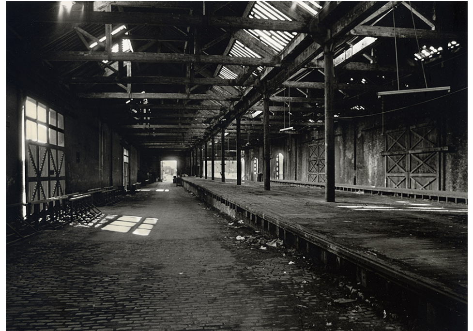
2.10 1978 view of Shipping Shed 1978 (Peter Fallas)
