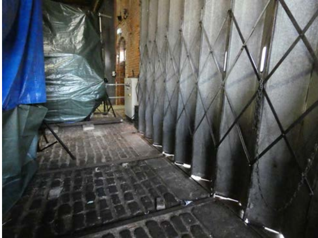
A.16 Railway entrance in the west elevation (Insal).
