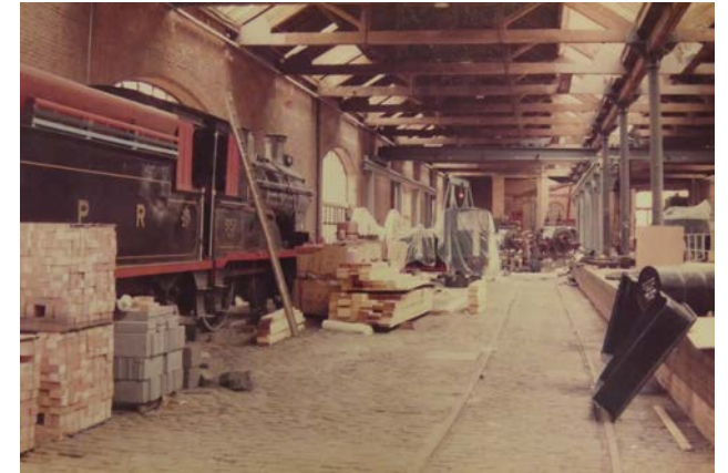
2.19 c.1983 View of the Power Hall (SIM Archive YA2007.4129. Licence CC-BY-NC-SA 4.0)
