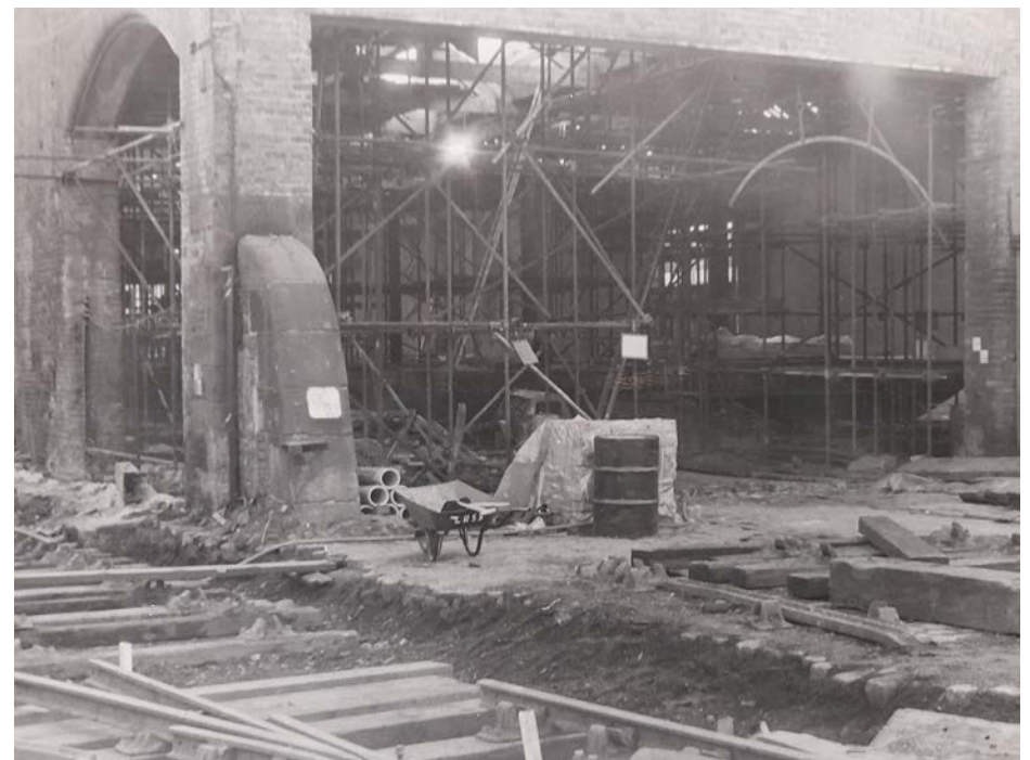
2.15 West end of Power Hall, 1979-80 (SIM Archive 1996.1539219. Licence CC-BY-NC-SA 4.0)
