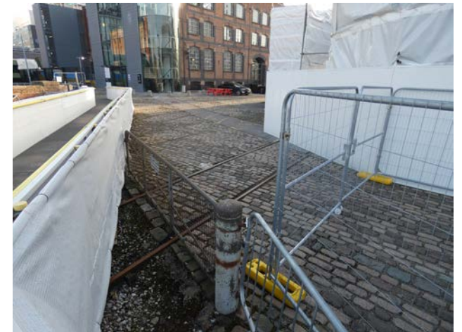
A.6 Setts in the Upper Yard, west end of Power Hall (Insal).
