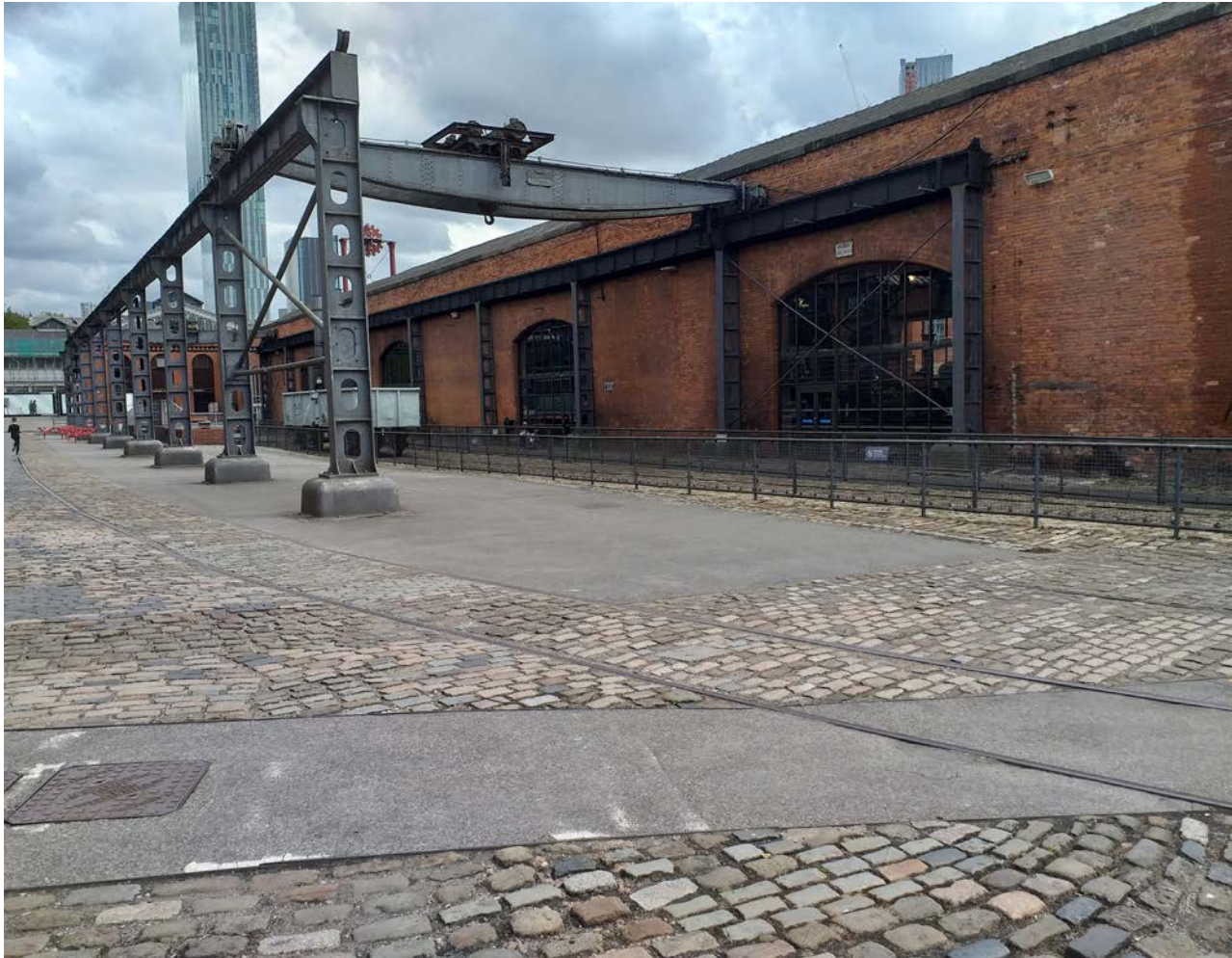
A.4 The Upper Yard to the north of the Power Hall (Studio Downie).
