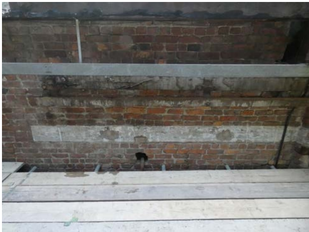
A.26 Iron runner and limewash above the east opening (Insall).
