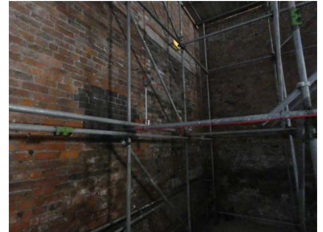
A.23 Blocked opening at the north-east corner (Insall).
