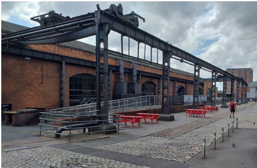
A.11 The Power Hall from the north (Studio Downie).
