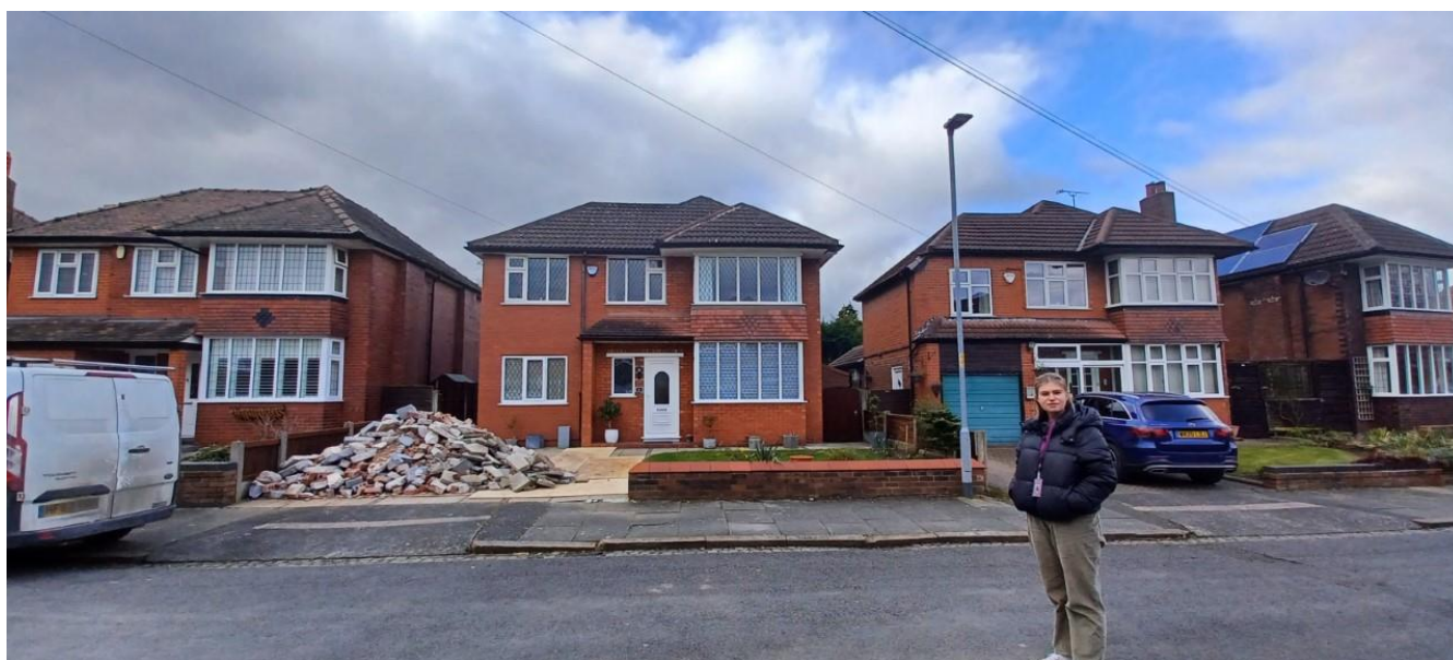
Figure 1. Principal elevation of No.6 Emsworth Drive.
