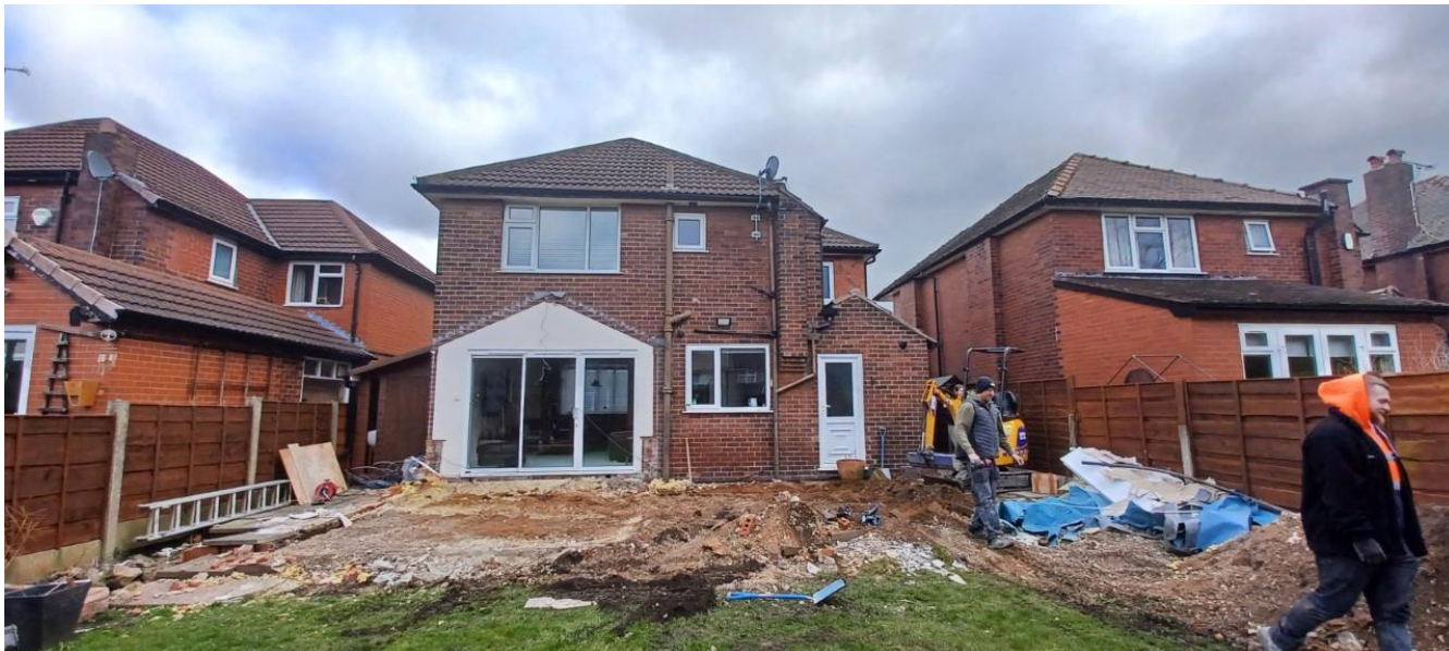
Figure 2. Rear view of the property.
