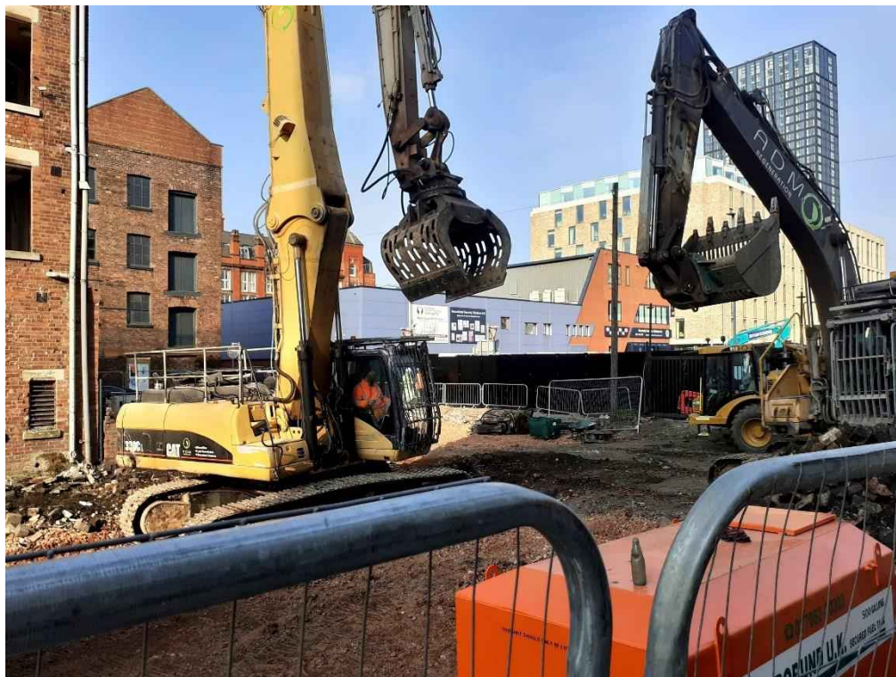
PLATE 4 TURNOVER OF MADE GROUND AND SORTING OF OVERSIZED MATERIAL
