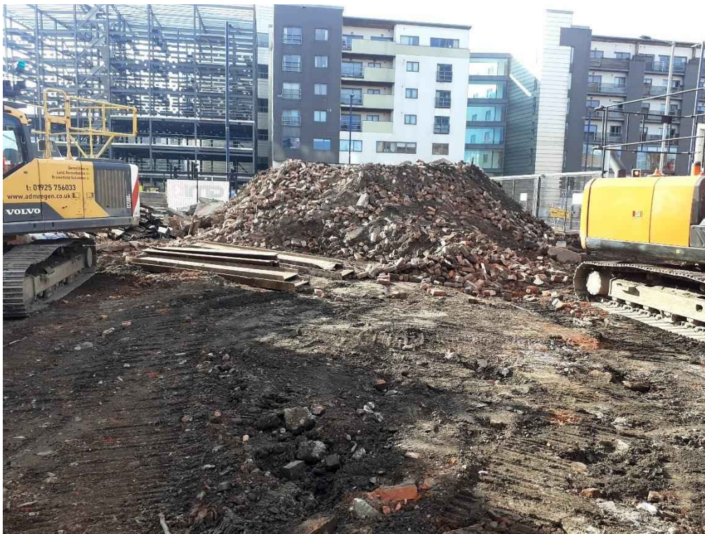
PLATE 6 STOCKPILE OF OVERSIZE MATERIAL AWAITING PROCESSING
