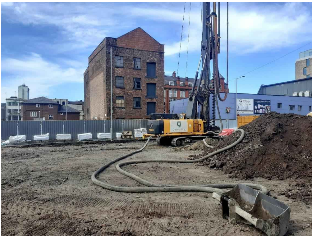
PLATE 10 VIEW OF SITE FACING WEST AND COMMENCEMENT OF PILING
