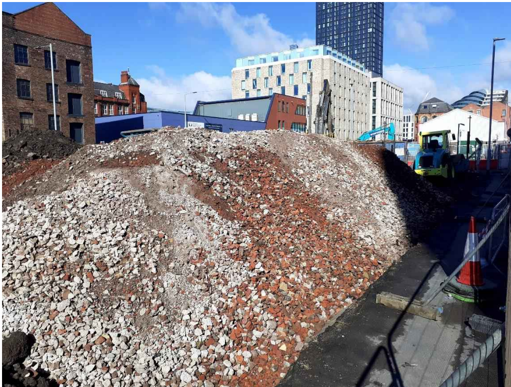
PLATE 7 STOCKPILE OF PROCESSED CRUSH
