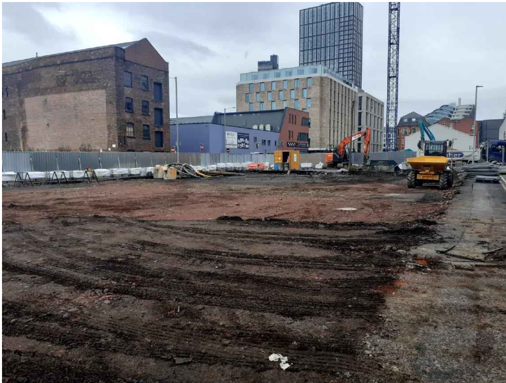
PLATE 9 VIEW OF SITE FACING NORTH
