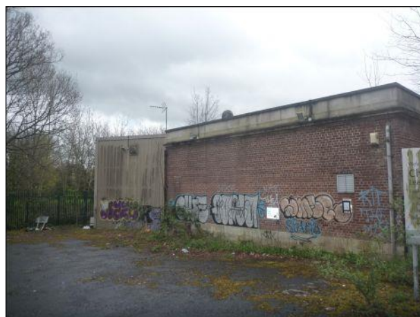
Photo 8: Building 1, northern elevation, western end
