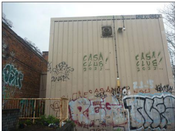
Photo 11: Building 1, showing southern elevation of metal extension
