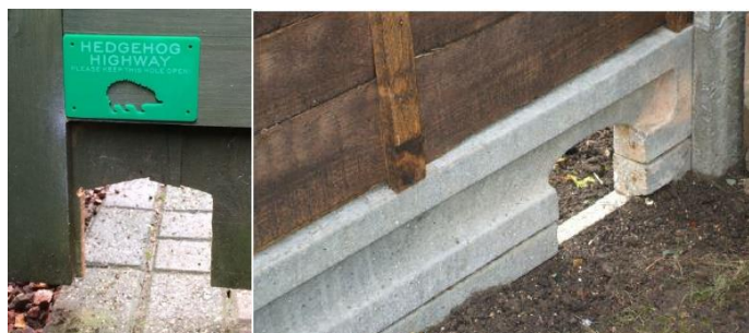
Insert 4: Showing wildlife access gap within fencing
