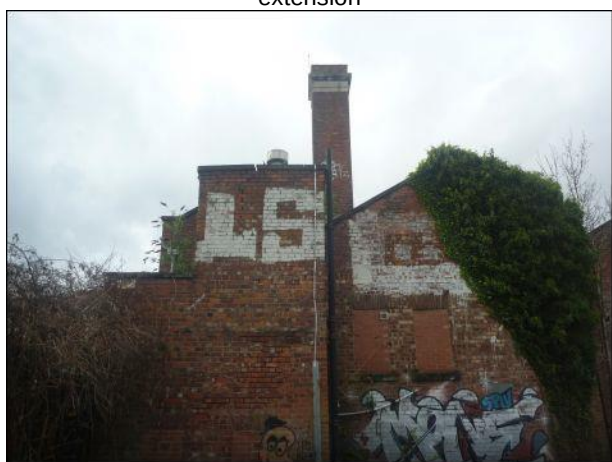
Photo 13: Building 1, south-eastern corner
