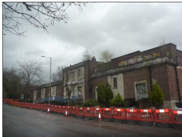
Photo 6: Building 1, western elevation, southern end
