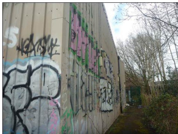
Photo 10: Building 1, eastern elevation, northern end
