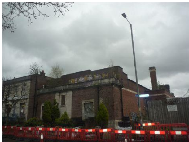
Photo 5: Building 1, south-western corner
