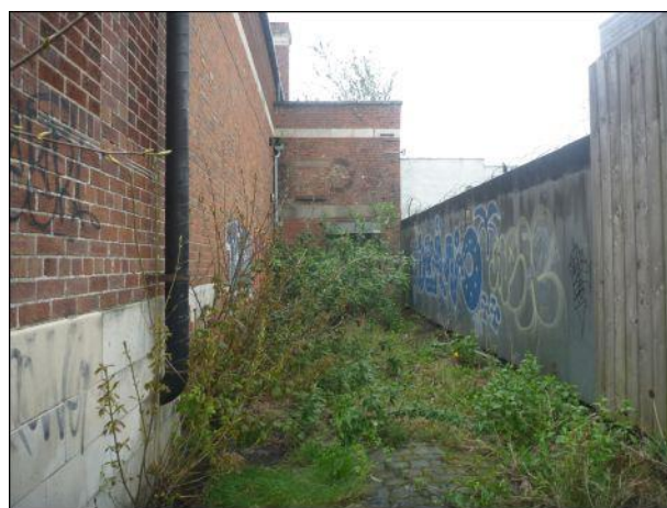
Photo 14: Building 1, south-western corner
