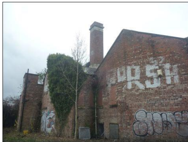
Photo 12: Building 1, eastern elevation, southern end
