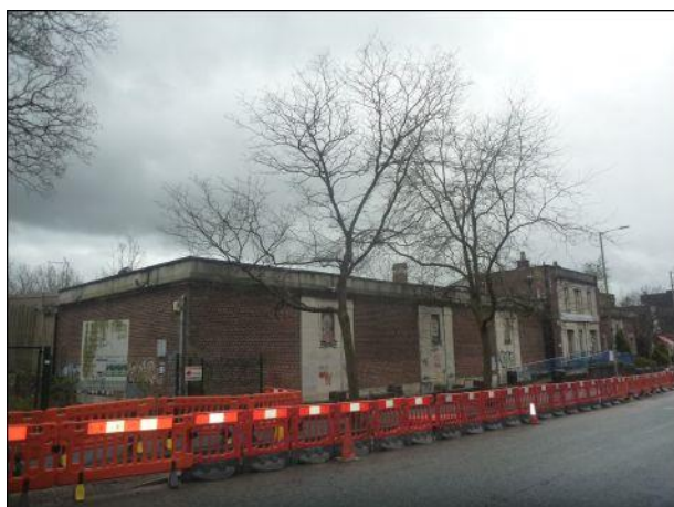
Photo 7: Building 1, western elevation, northern end
