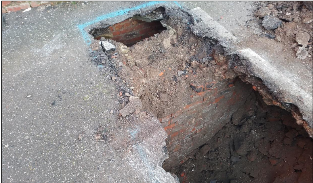
Plate 5: Wall 103 in trench1, looking north
