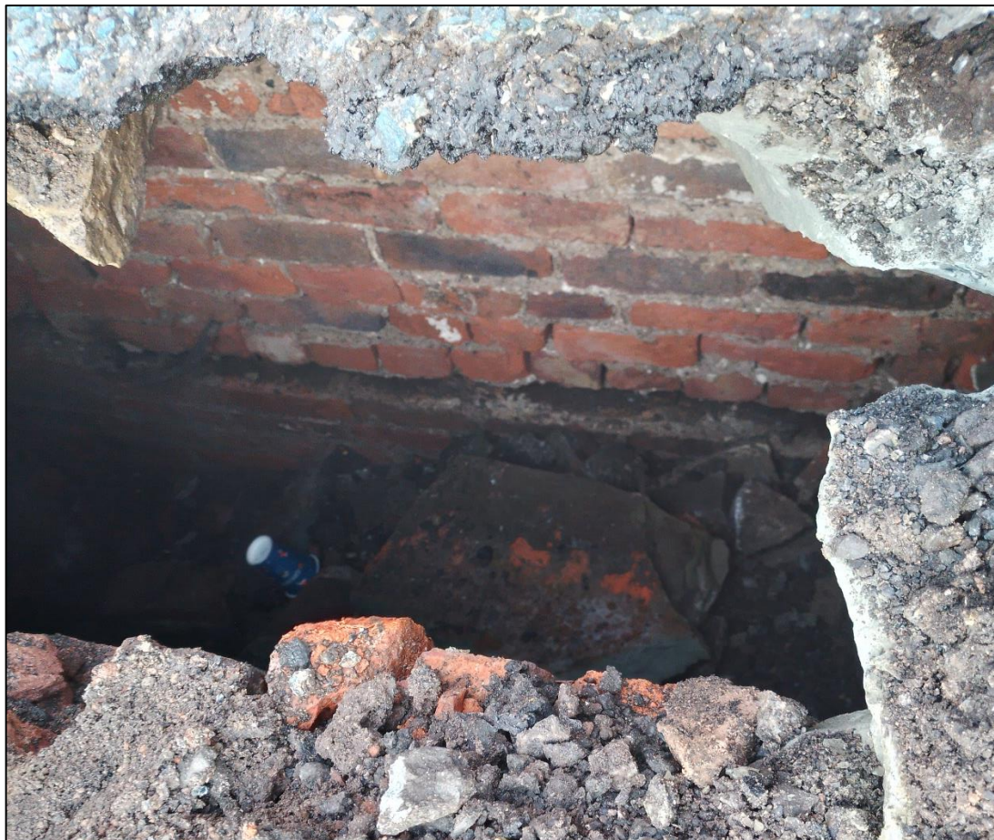
Plate 6: Wall 106 and associated void, looking northwest
