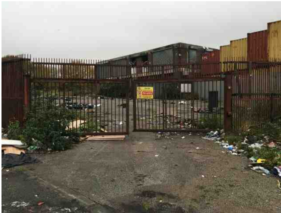
Photograph 1: View of the site access via Broughton Street.
