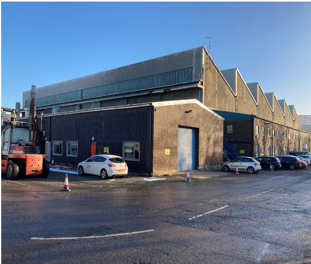
Picture 1 – Hangar 4 view facing east
