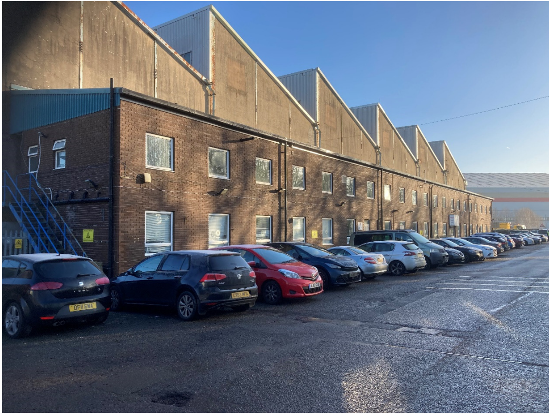
Picture 5 – 2 storey office building
