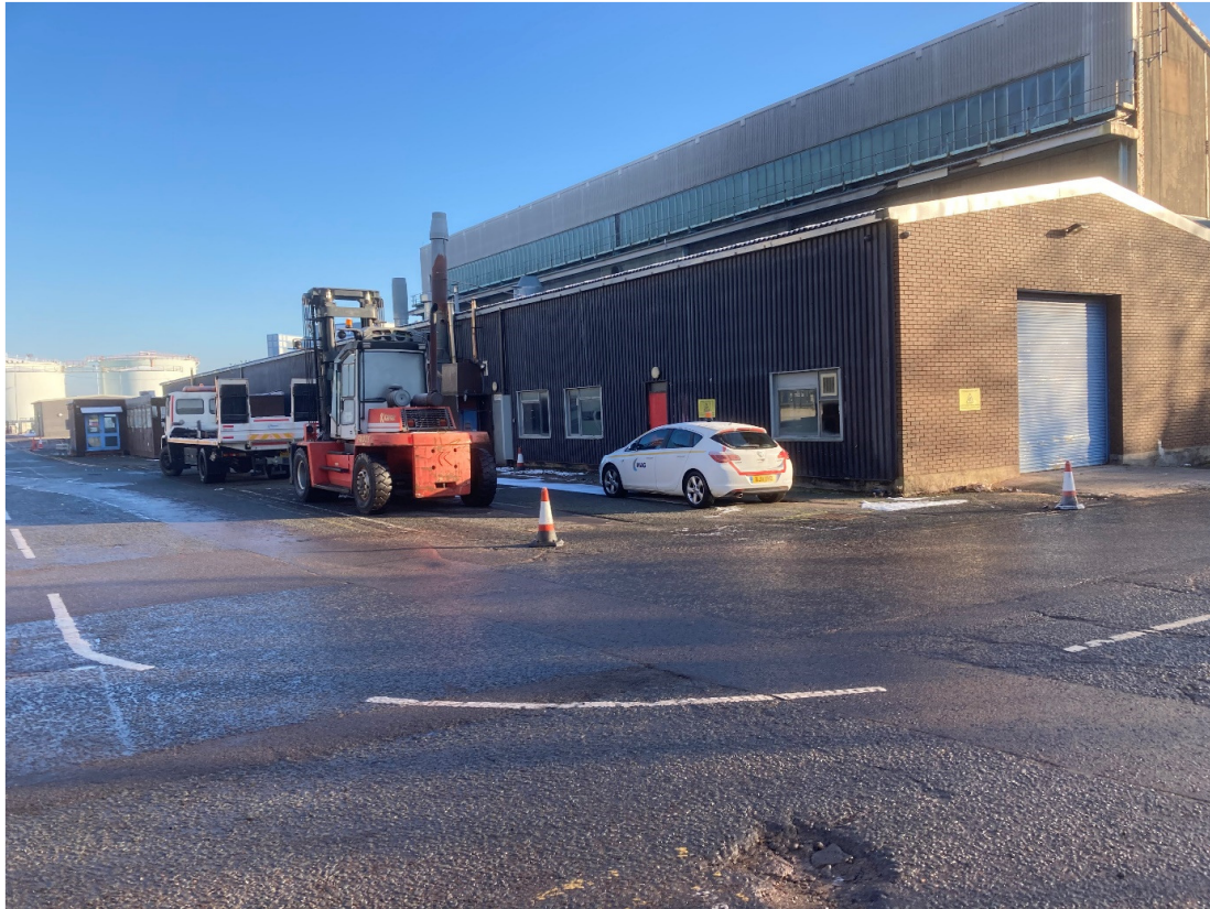
Picture 4 – North West Annex building showing fume extraction equipment behind the fork lift truck
