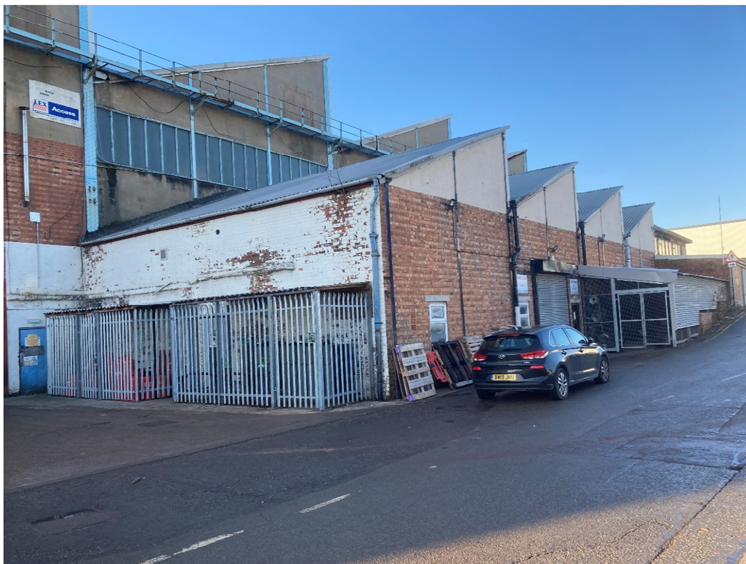
Picture 3 – North east extension to Hangar 4 building
