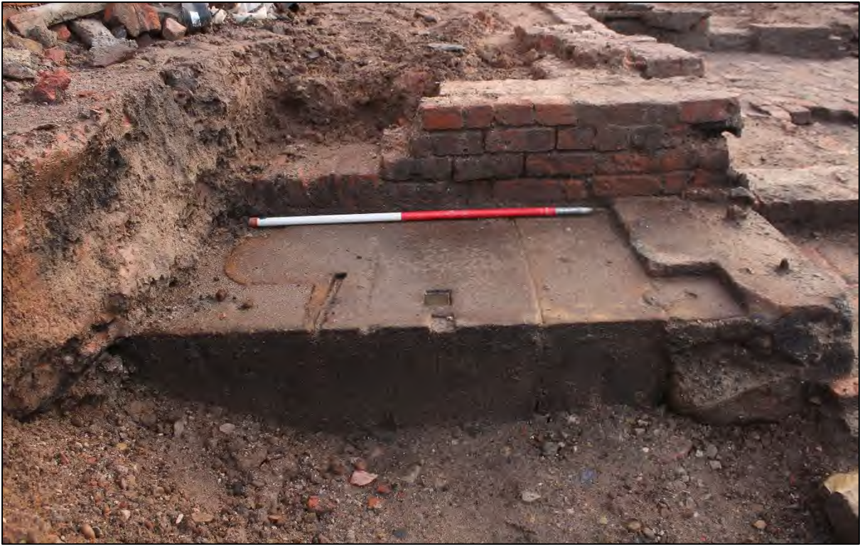
Plate _: View of the adjoining blocks making up engine bed 3140 (1m scale)
