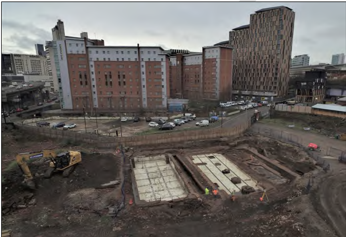
Plate xx: Aerial view of Mayfield Baths looking north-east
