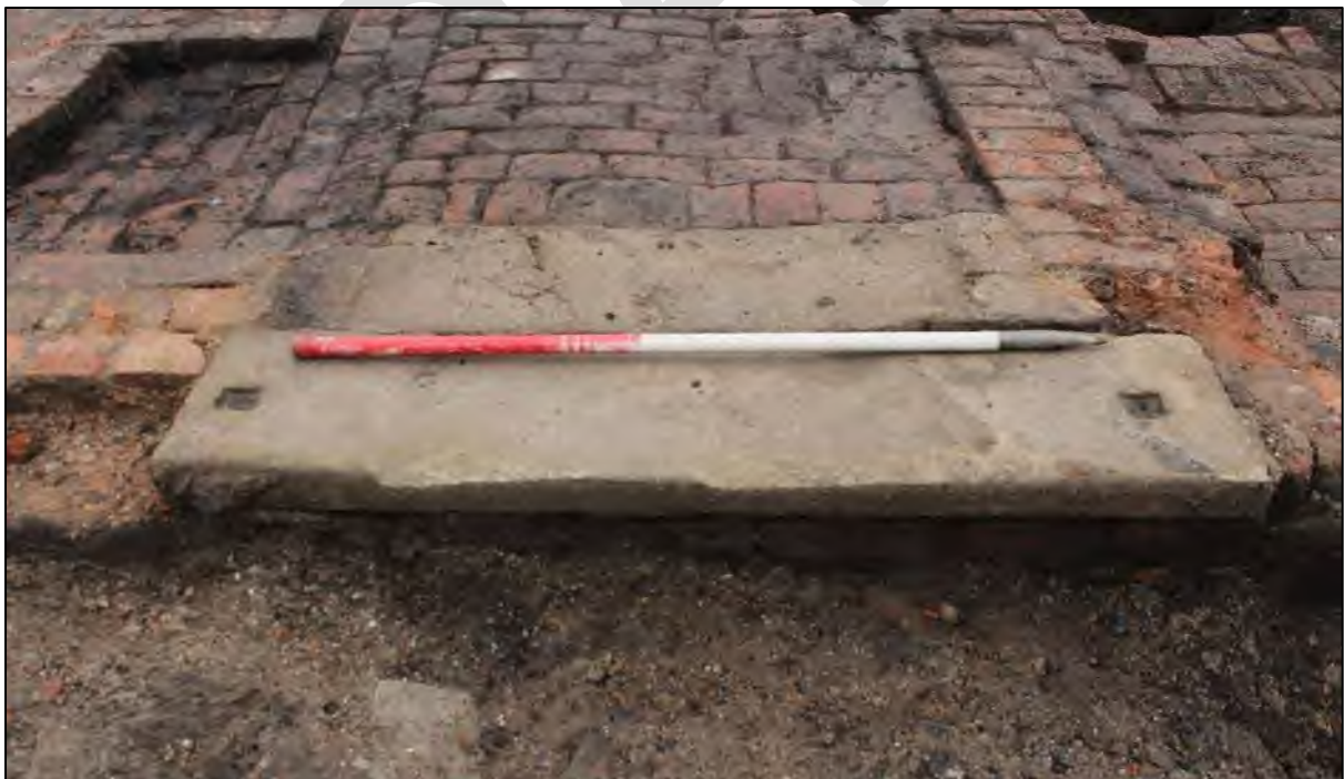
Plate_: Wall 3010 featuring a later threshold with rectangular sockets for the door jambs. The earlier wall and threshold are visible to the rear. Both exhibit traces of significant wear. (1m scale)
