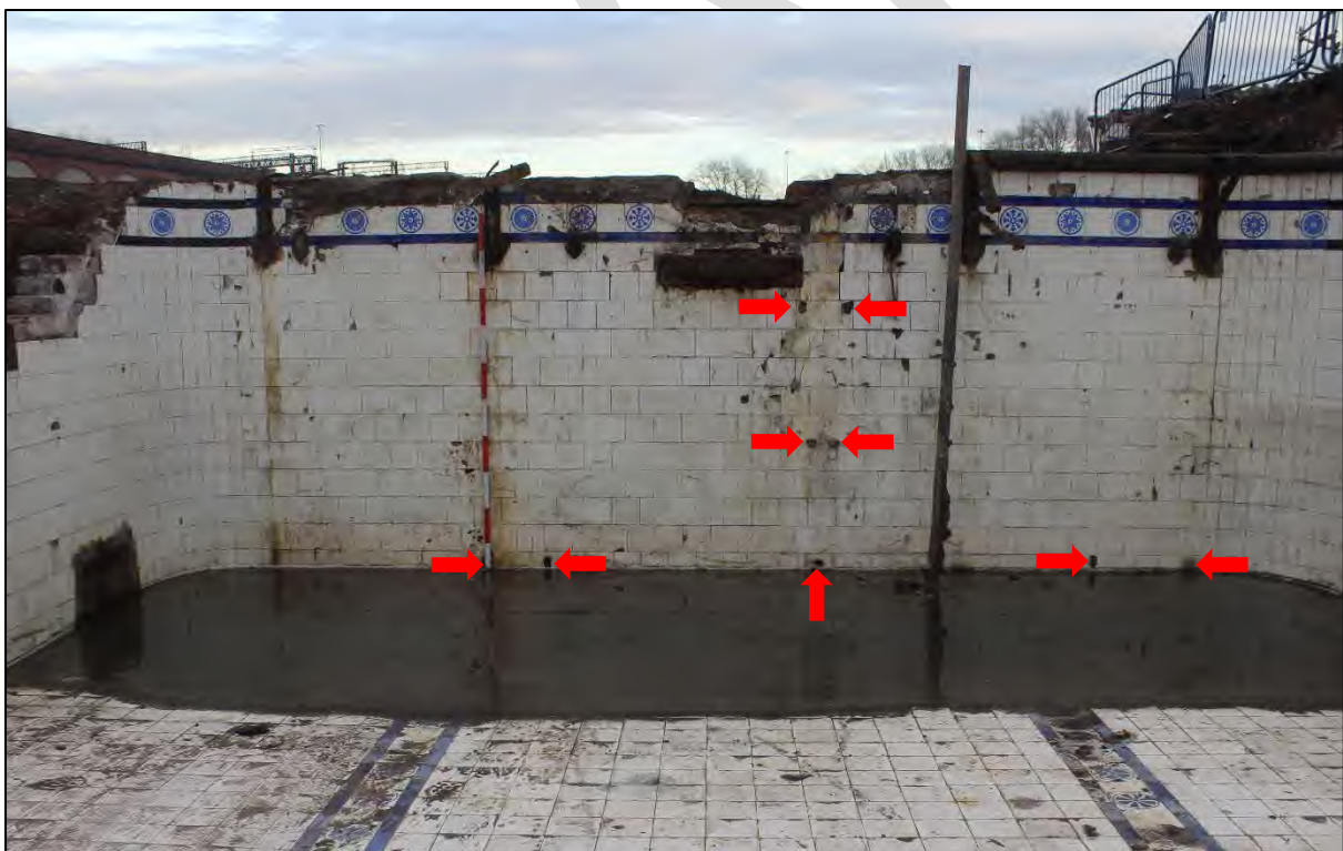
Plate xx: The eastern end of Pool 225 showing the position of the fixings for the steam injection pipe (removed) and L-shaped brackets visible above the waterline (2m scale)
