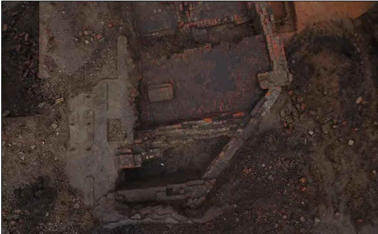
Plate x: Part of the Phase 5 extension to the south of the boiler house
