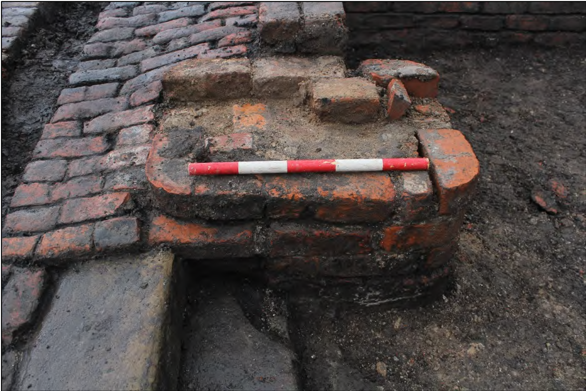
Plate_ : Detail of brick pier 3124 with adjacent surface 3168, looking south (0.50m scale)
