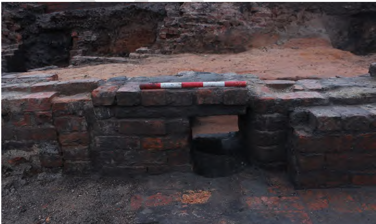
Plate 2: Western elevation of wall 3070 with blocked doorway 3191 (0.50m scale)
