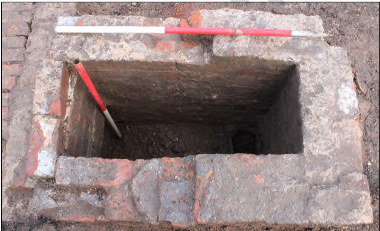
Plate_: View of the interior of chamber 3108, note the cast-iron plate on its southern side, looking east (2 x 1m scales)
