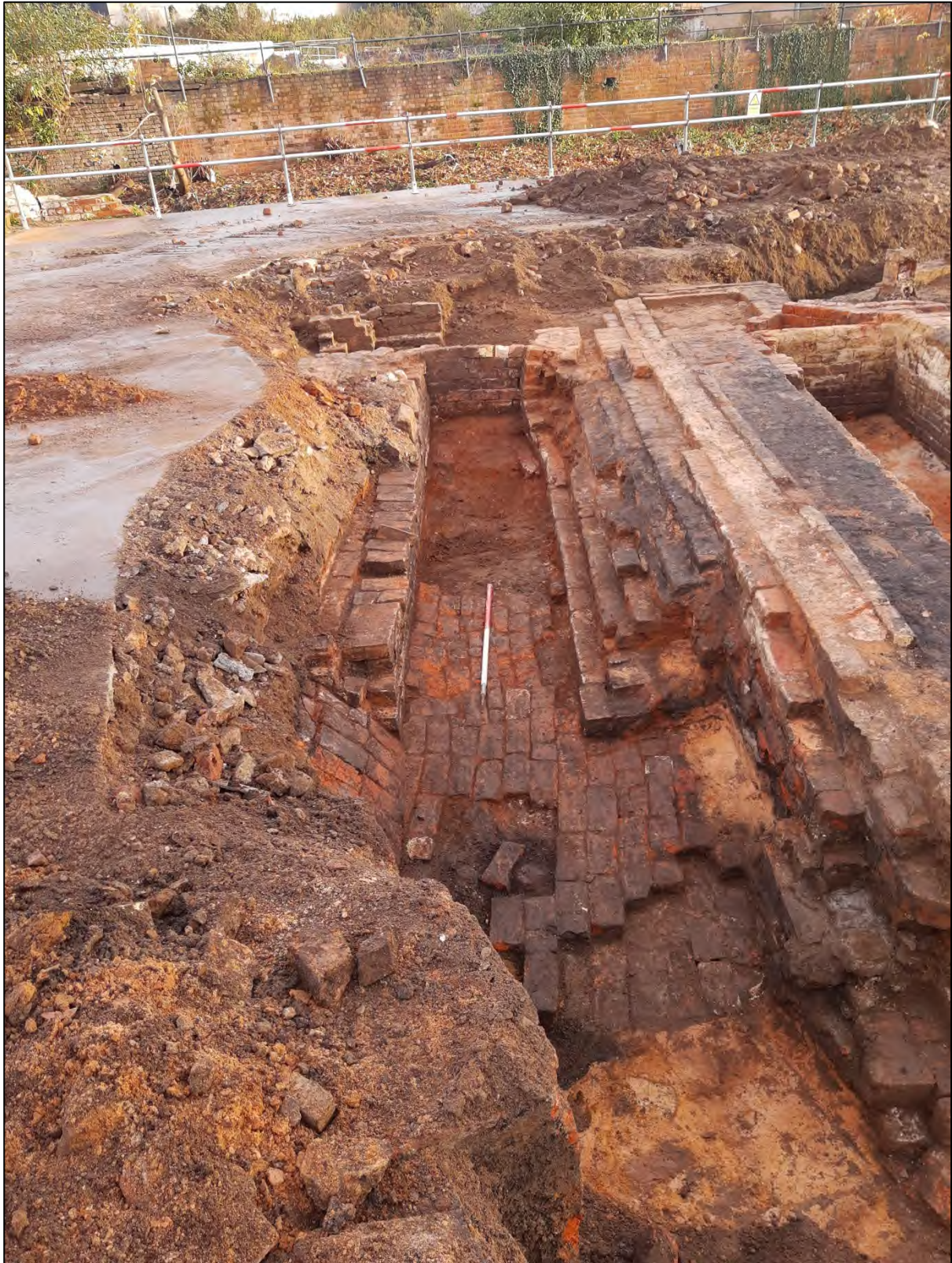
Plate xx: Boiler 112, looking north
