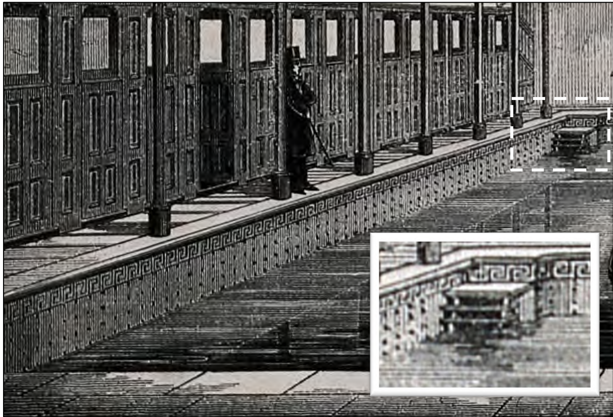
Plate x: Extract from The Builder 1858 showing the original tiles and steps installed in the plunge pool of the first-class men's pool at Mayfield Baths (see inset for close-up)
