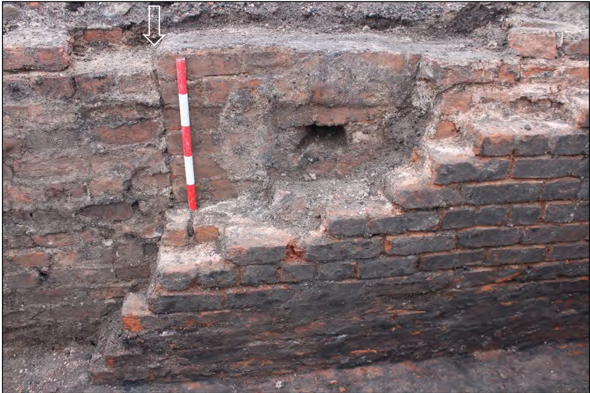
Plate_: Phase break between walls 3171 and 3178 with the western wall of walkway 3069 in the foreground, looking west (0.50m scale)
