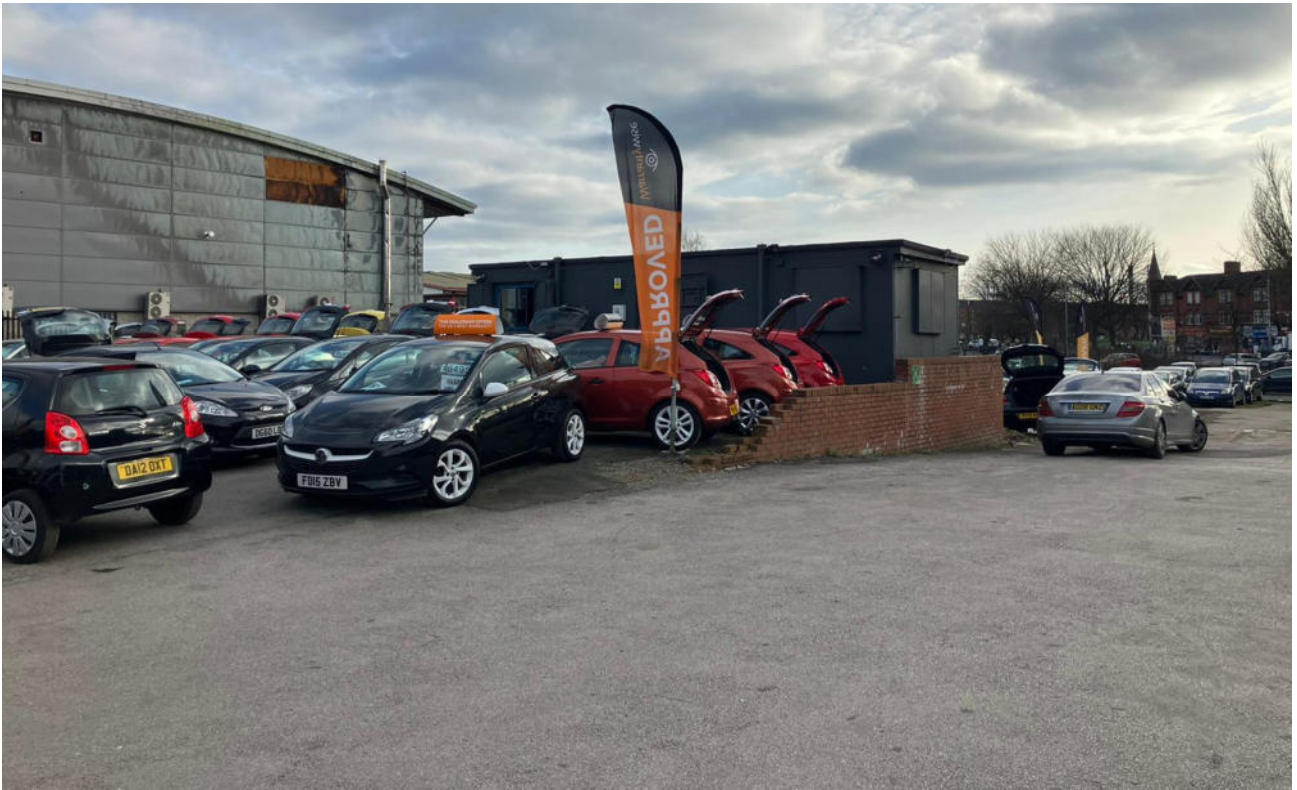
Photograph 1 - North east of the site and one of the commercial units currently present on site.
