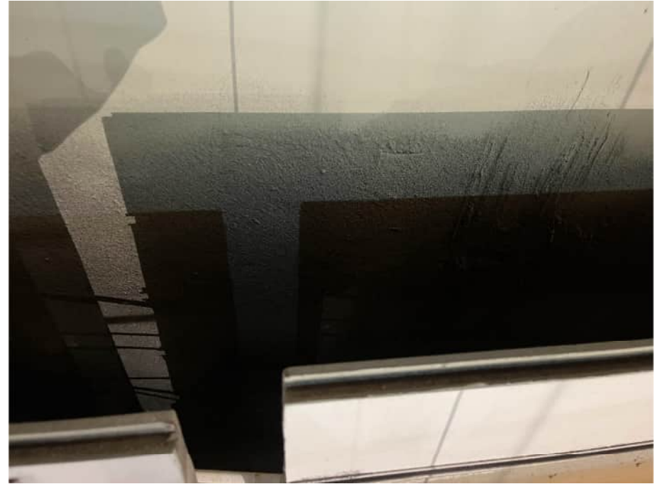
1. E (behind fit out 2)
