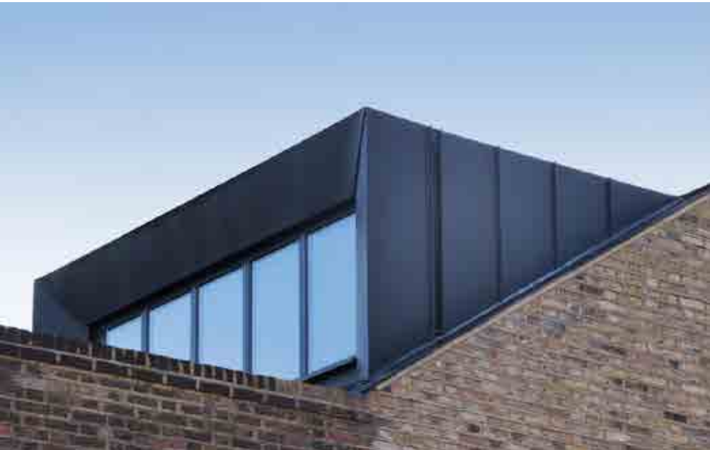
DORMERS - ZINC CLAD DORMER WINDOWS TO FRONT ELEVATIONS AT ROOF LEVEL
