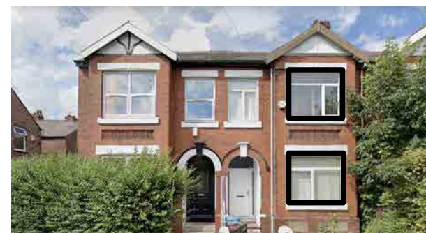
EXISTING TERRACE ON BERKELEY AVENUE
