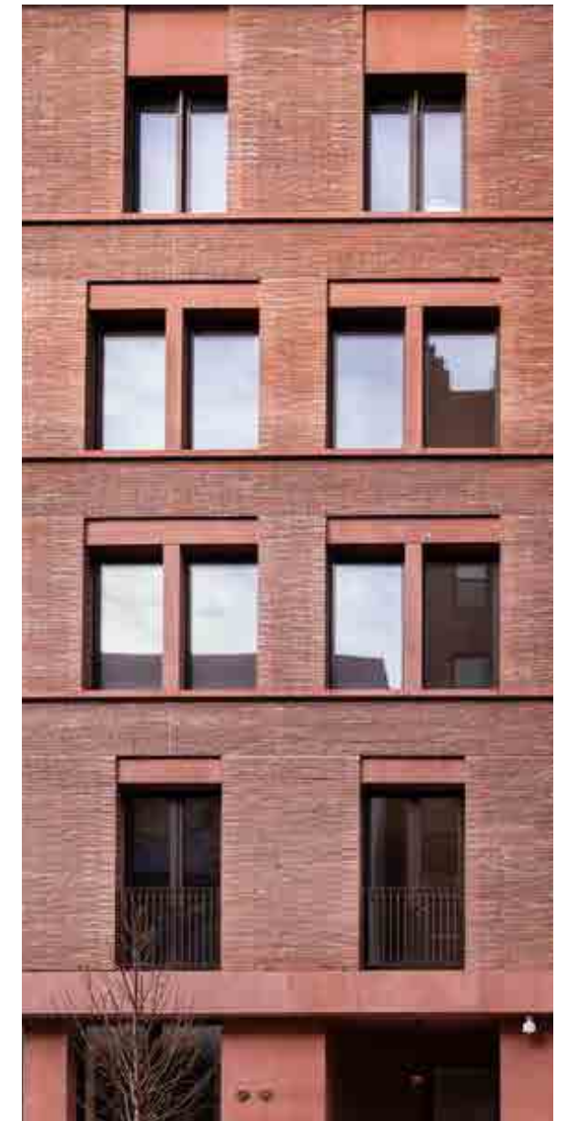
RECESSED WINDOW HEAD DETAIL
