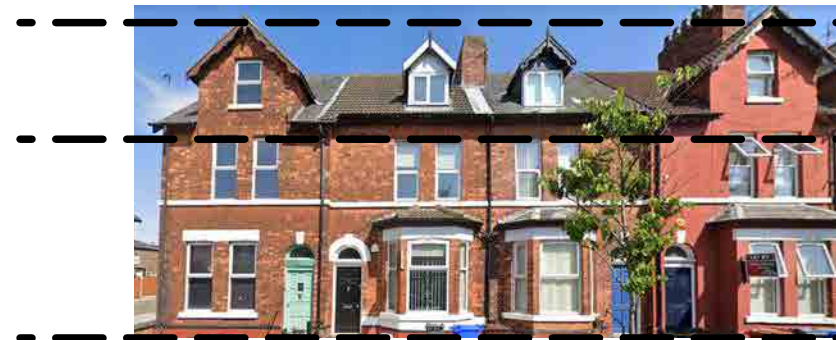
EXISTING TERRACE ON LONGFORD PLACE
