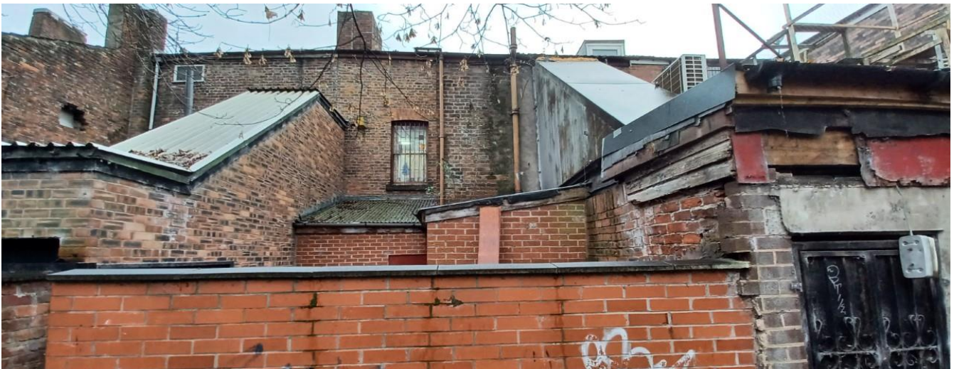
Figure 2. Photograph depicting the existing single storey rear extensions at the property.
