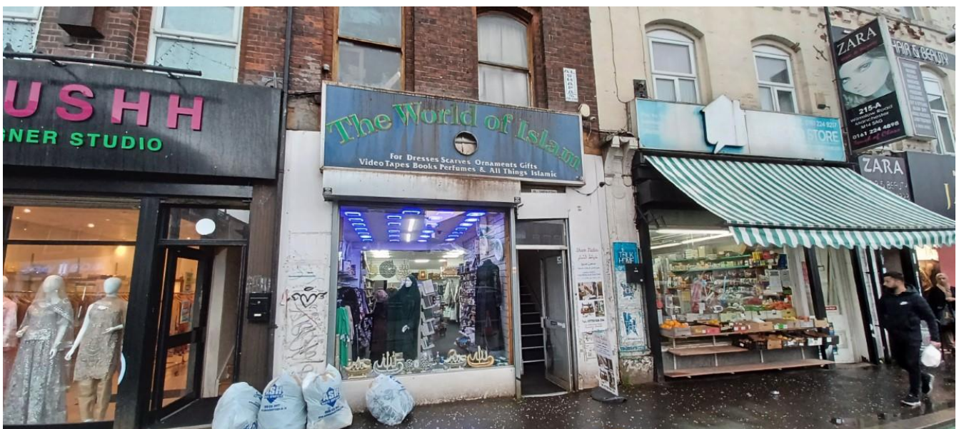
Figure 1. Photograph of the principal elevation of No.211 Wilmslow Road.
