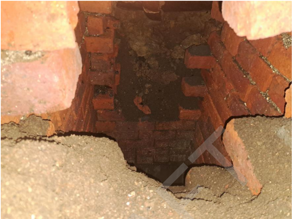
Plate 7 - Trench 2. Brick chute below platform 201
