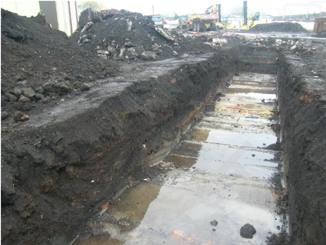
Plate 19 - Trench 8. Overview of trench, looking south-east
