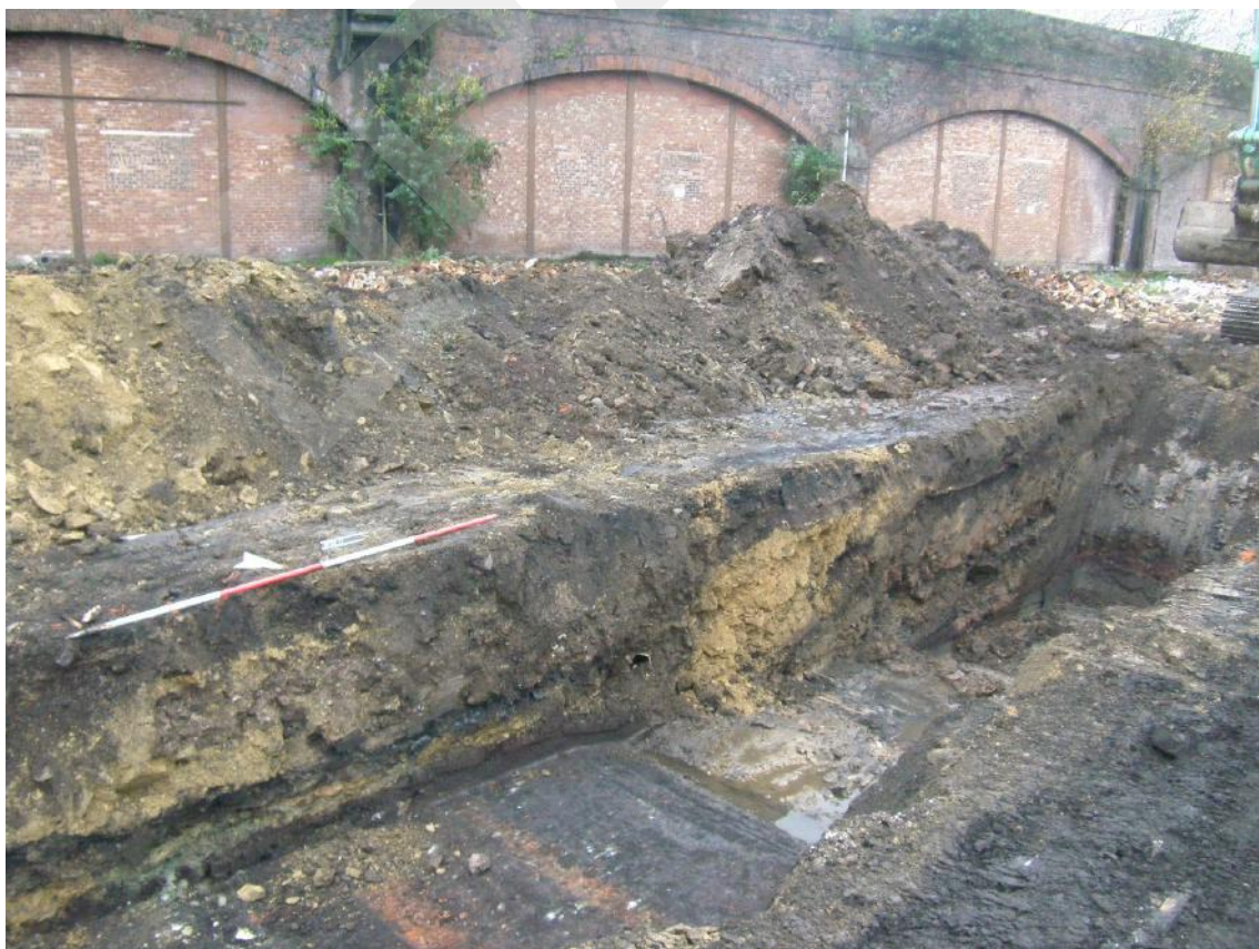
Plate 18 - Trench 7. North-east facing section showing loose sand deposit 708, sleeper 704, cinder surface 706, potential wall foot
