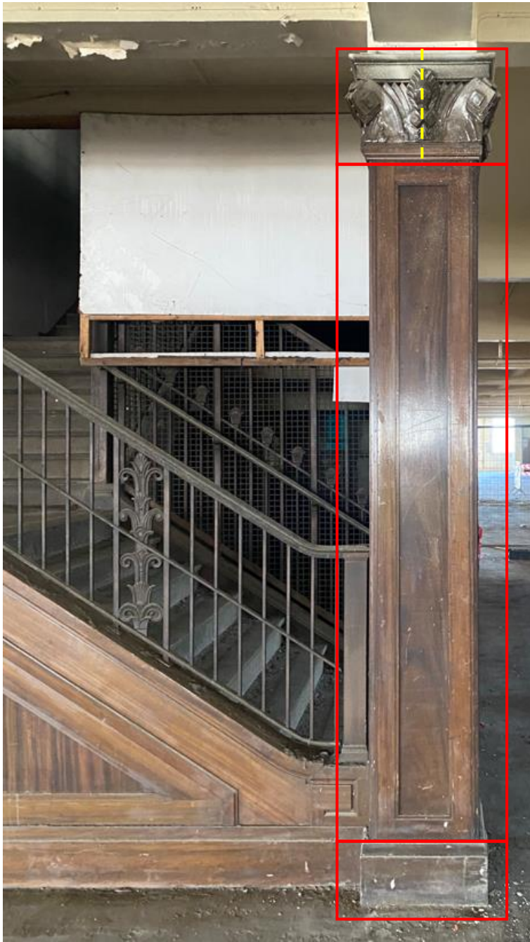
Figure 10 – Column encasement removal
