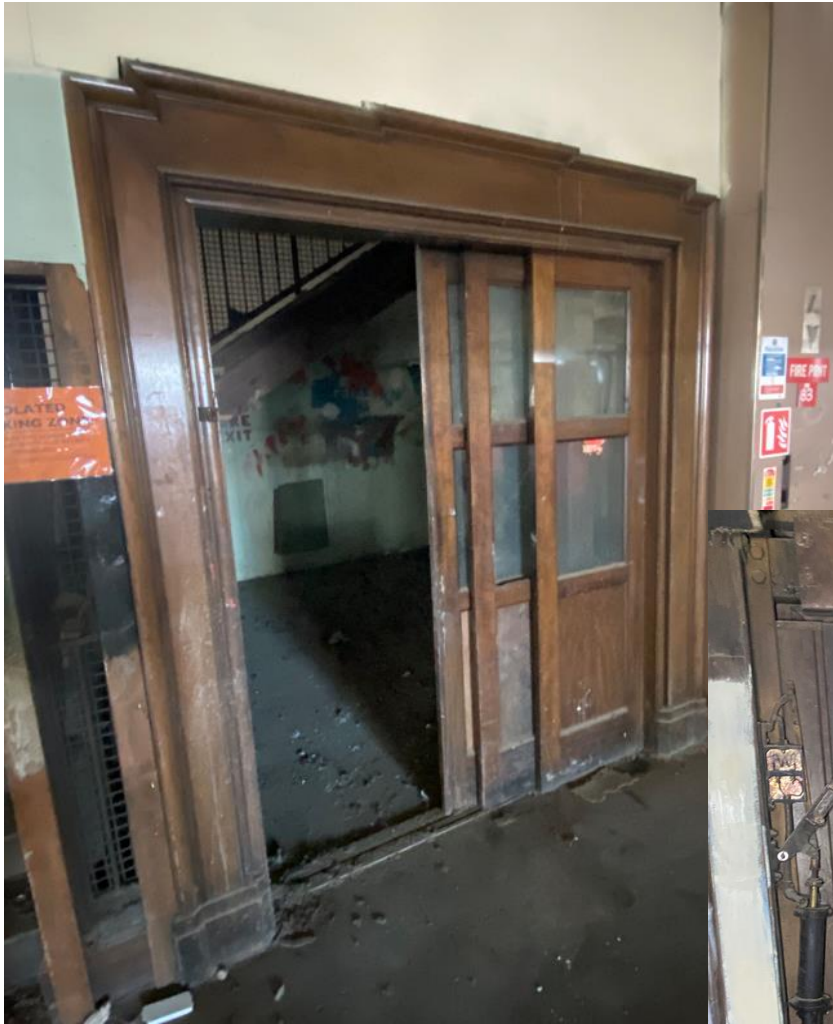
Figure 12 – Lift door removal
