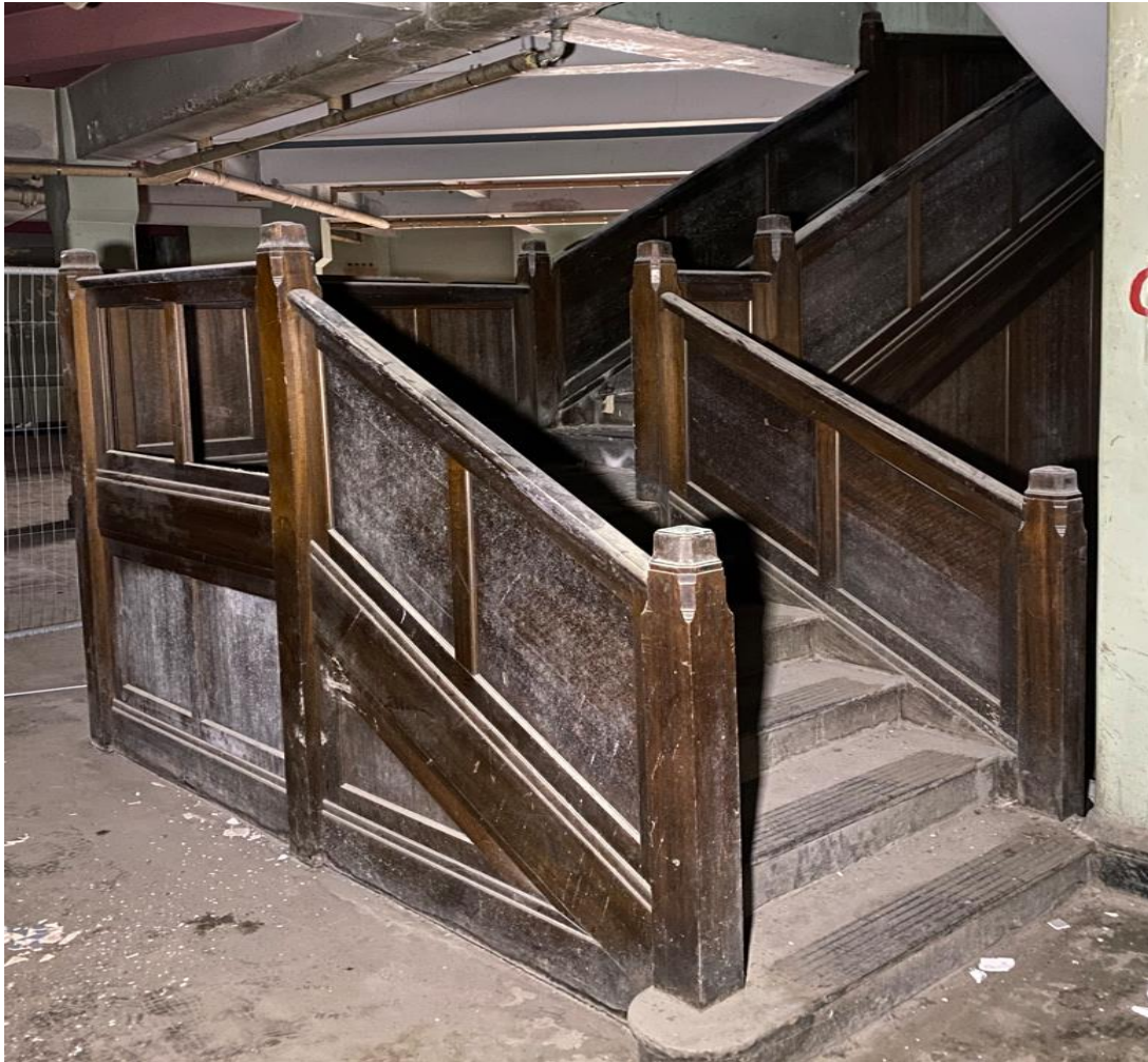
Figure 16 – Heritage Staircase 2 removal
