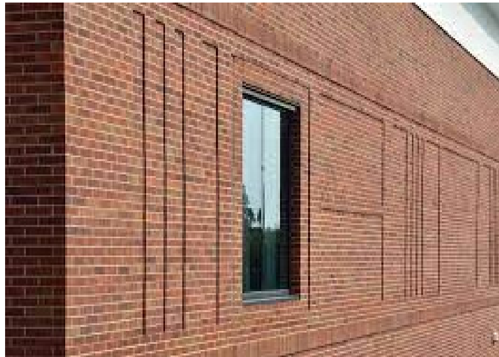
RECESSED BRICKWORK PANEL
