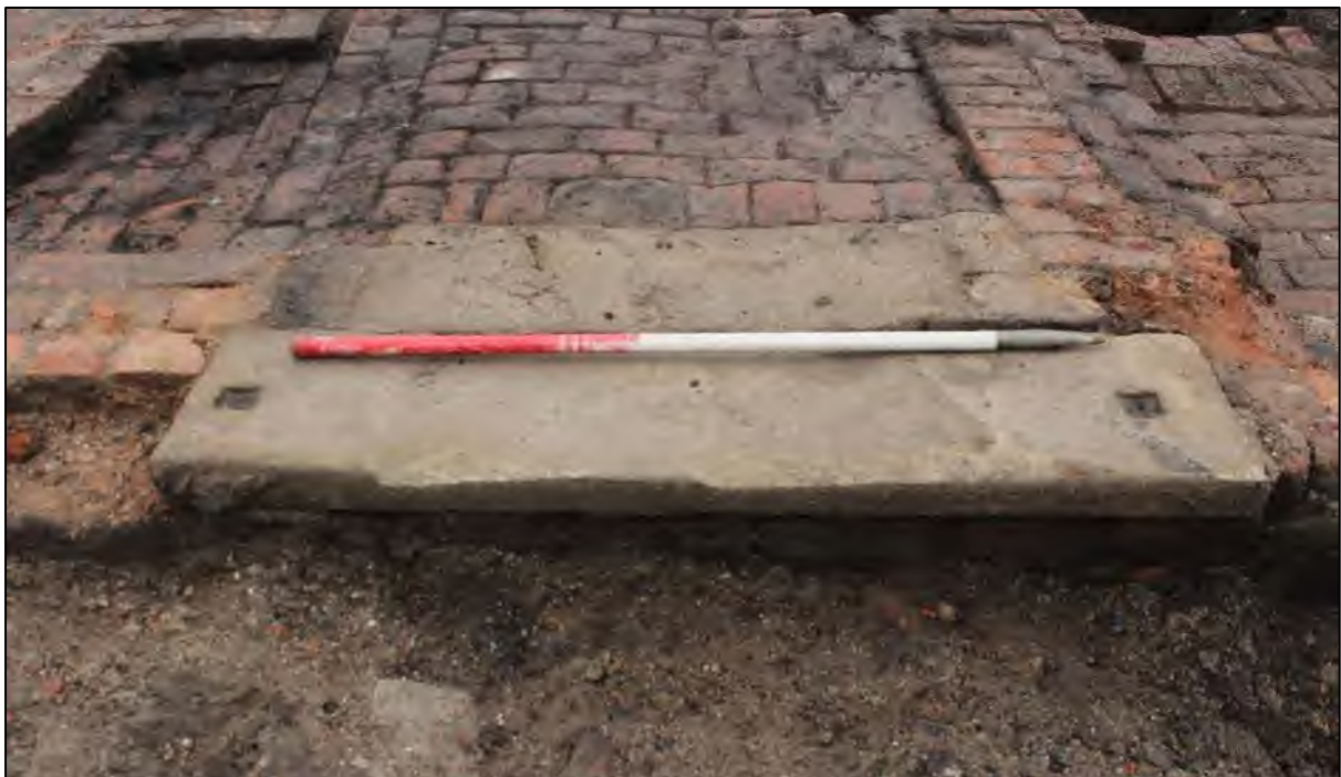
Plate 83: Wall 3010 featuring a later threshold with rectangular sockets for the door jambs. The earlier wall and threshold are visible to the rear. Both exhibit traces of significant wear. (1m scale)
