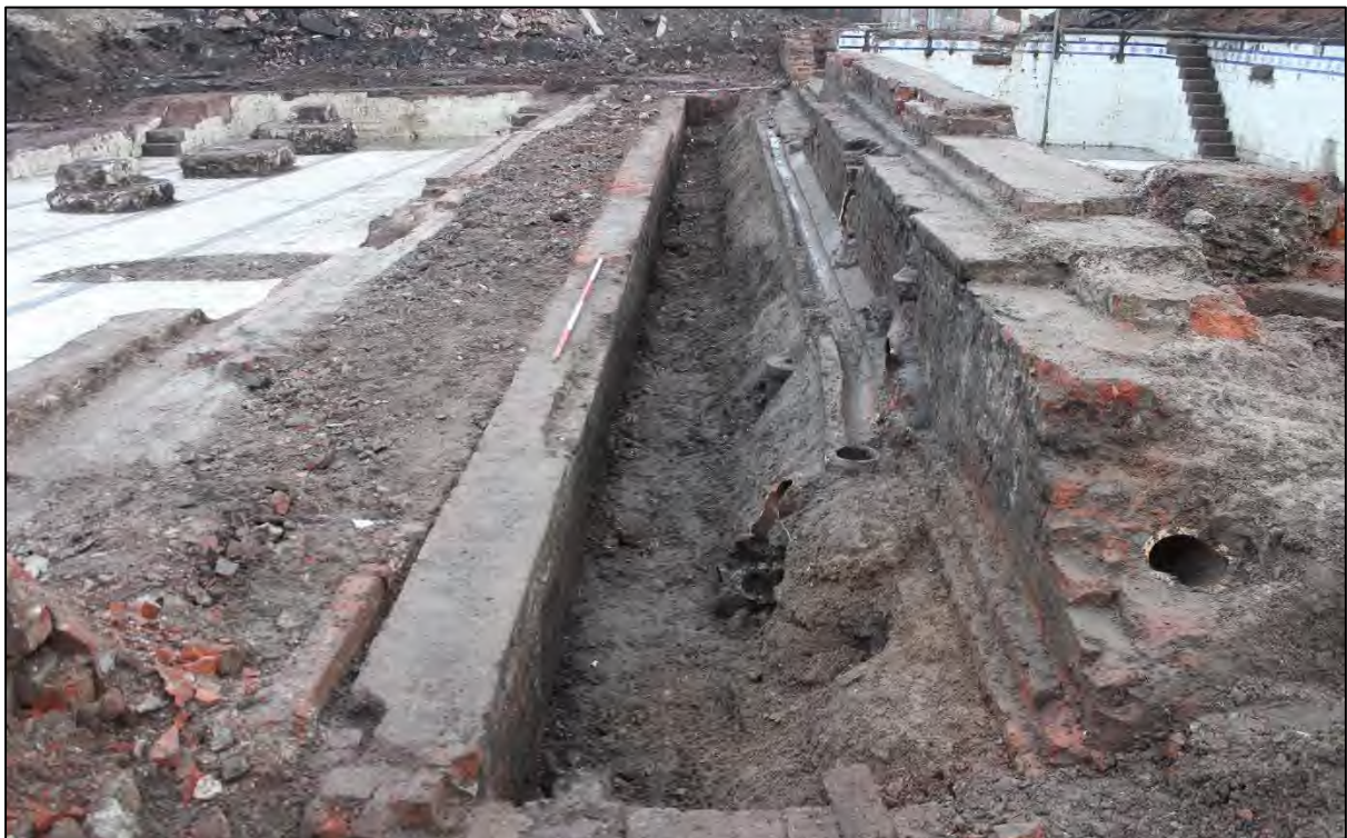
Plate 48: Wall 227 looking east
