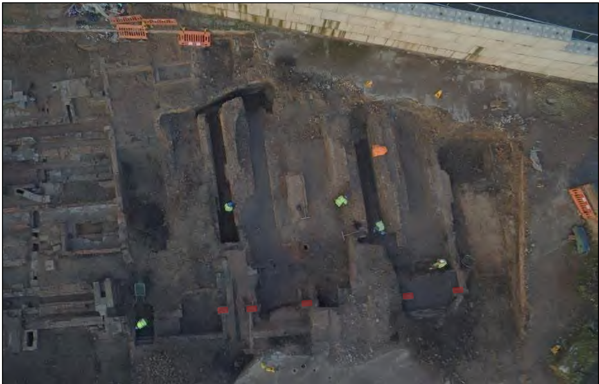
Plate 127: Aerial view of the boiler House undergoing excavation with the brick piers forming the southern side of the building in Phase 3 highlighted (red)
