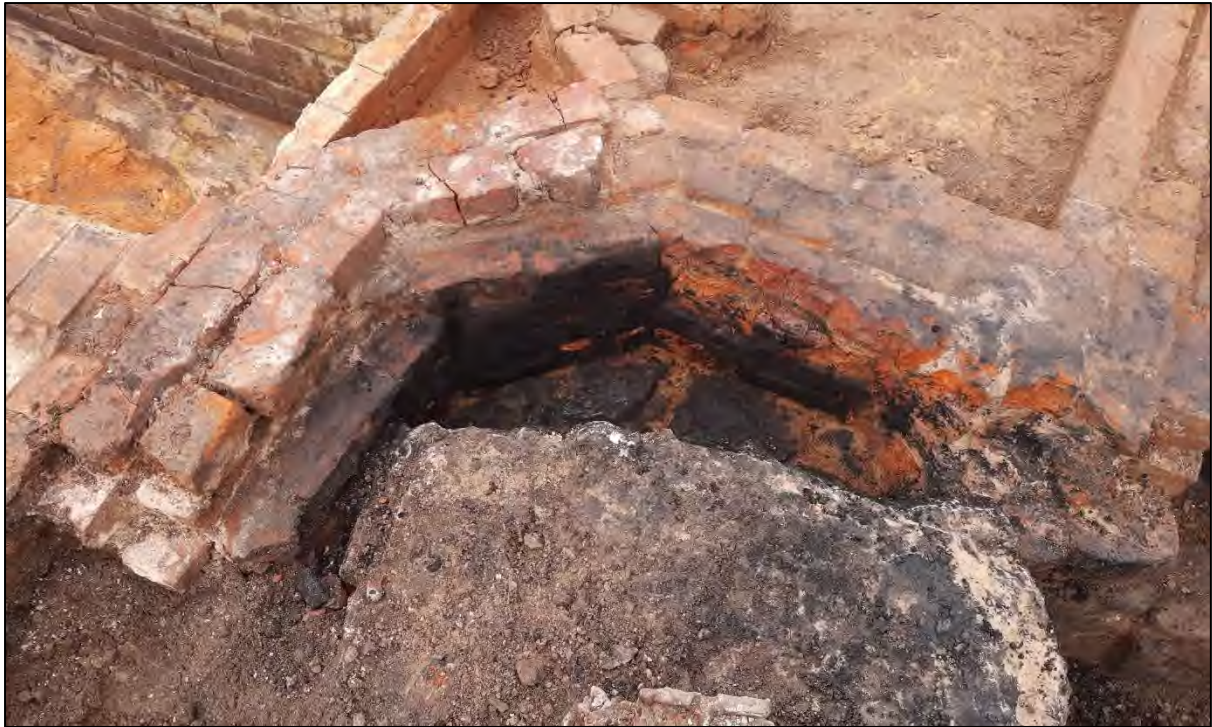
Plate 42: Chimney structure 110, looking west.
