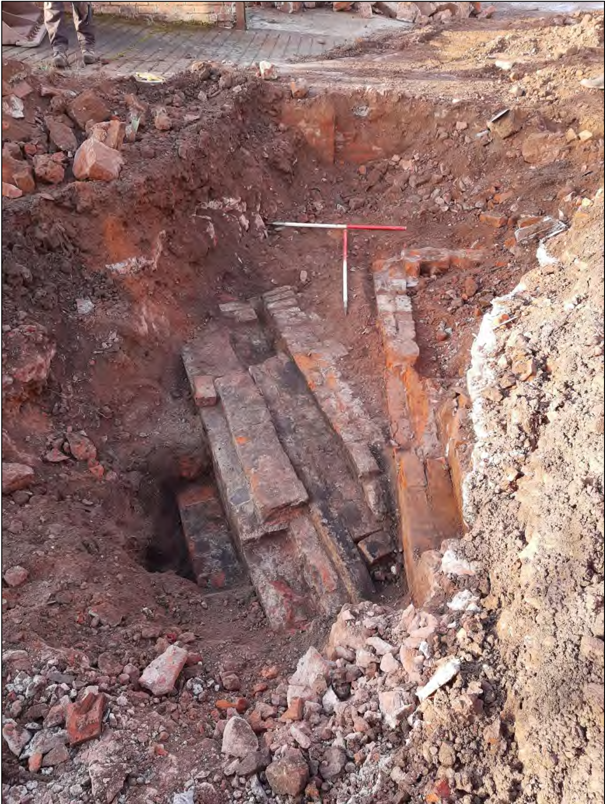
Plate 31: Trench 7, looking southwest.
