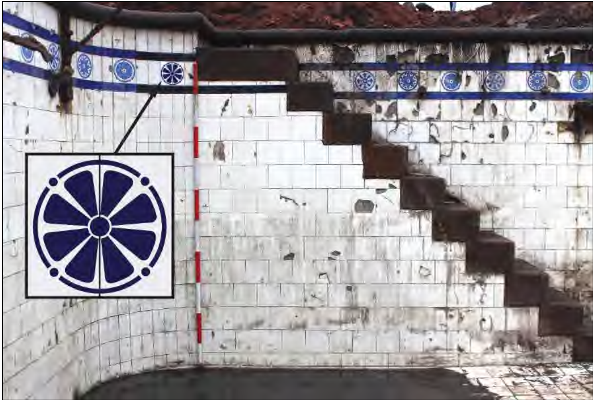
Plate 61: Pool 225 showing the later steps and replacement tiles (2m scale)
