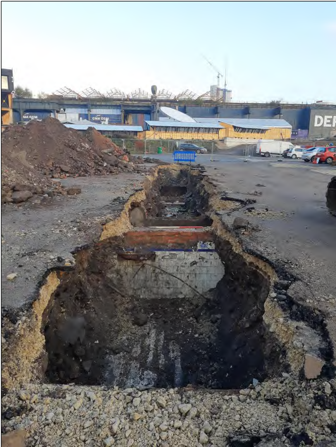
Plate 32: Trench 8, looking north.
