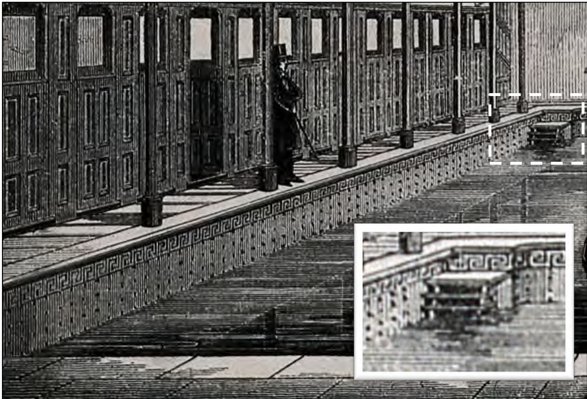
Plate 187: Extract from The Builder 1858 showing the original tiles and steps installed in the plunge pool of the first-class men's pool at Mayfield Baths (see inset for close-up)
