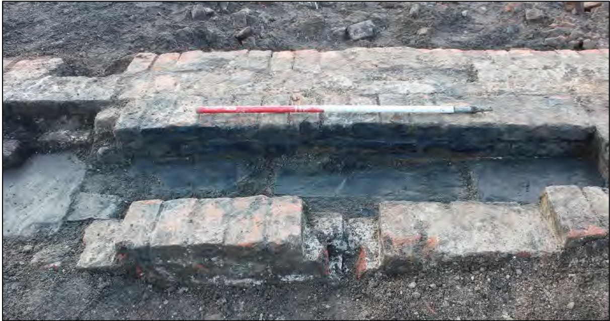
Plate 81: Slate-lined drain 3039 (1m scale)
