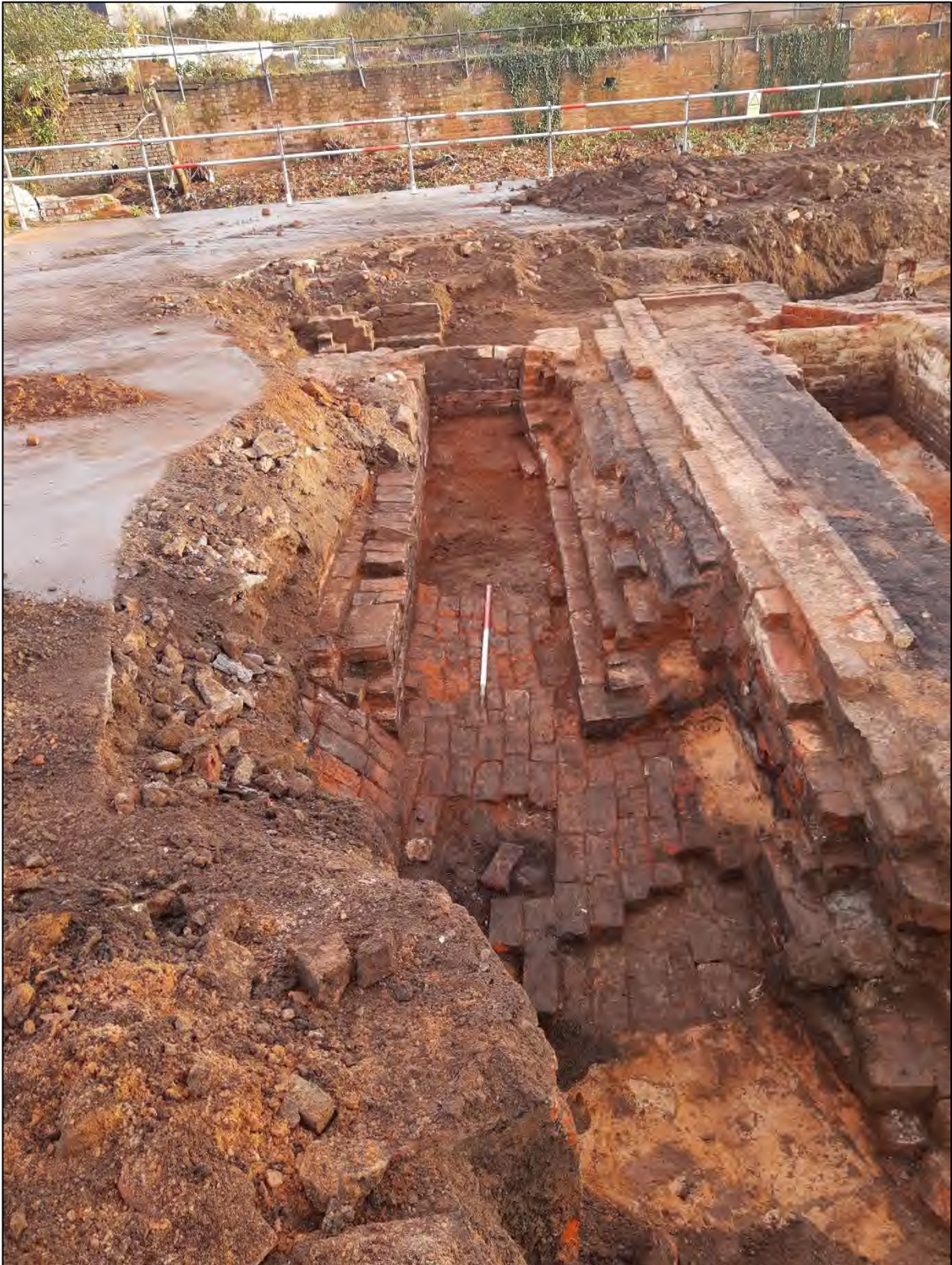
Plate 45: Boiler 112, looking north (1m scale)
