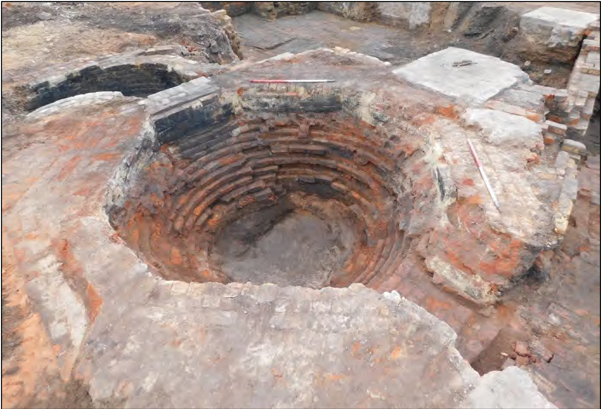
Plate 162: Chimney 424, facing south east (2 x 1m scales)
