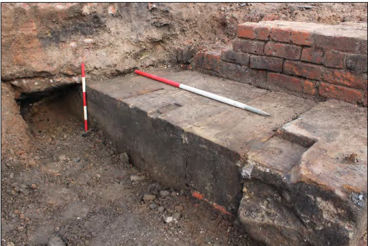
Plate 111: View of the adjoining blocks making up engine bed 3140 (0.50 and 1m scales)
