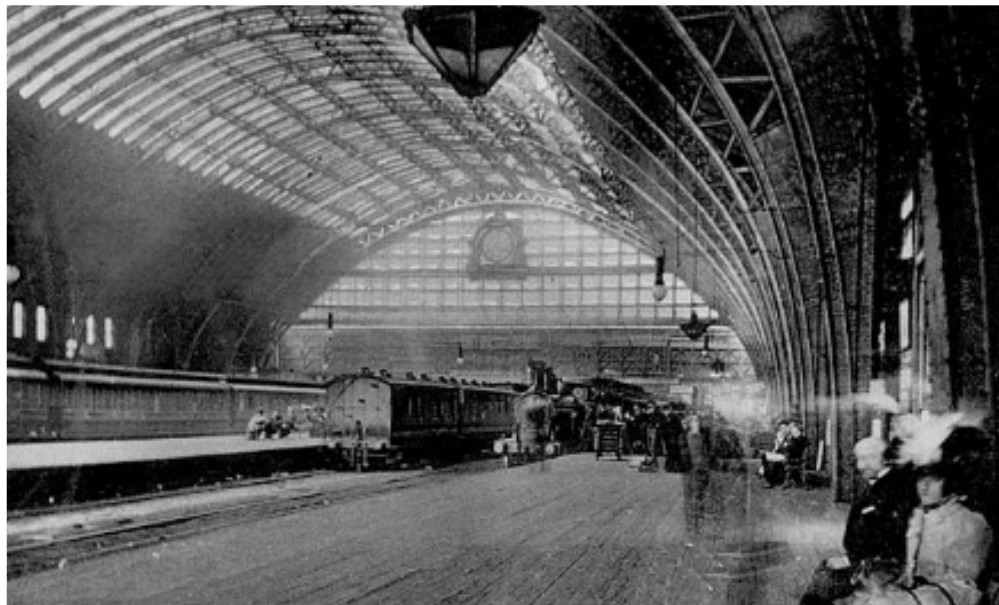
Internal view of the train station in the first decade of the 20 th century (image John Alsop collection)
