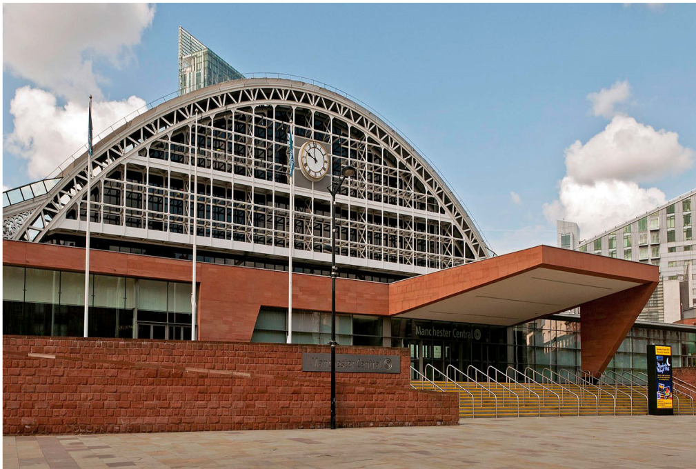
Views of front façade Stephenson Bell extension (Image Manchester Central)
