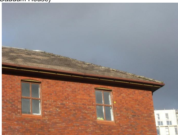
Photo 10: Showing slate roof and clay ridge tiles at Building 1 (Gaddum House)
