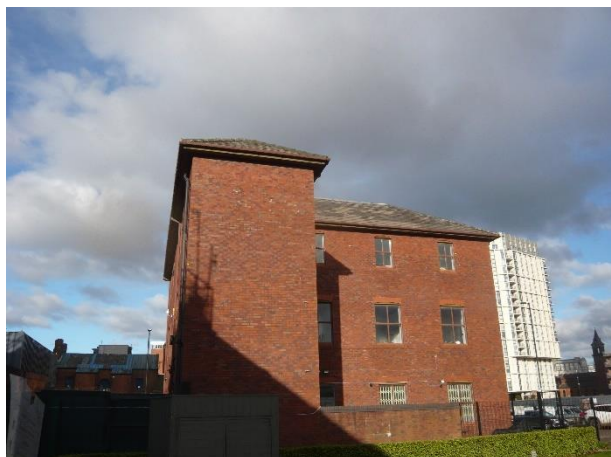
Photo 7: South-eastern elevation of Building 1 (Gaddum House)
