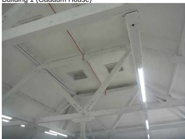
Photo 11: Showing underside of vaulted ceiling and roof beam structure, Building 1 (Gaddum House)
