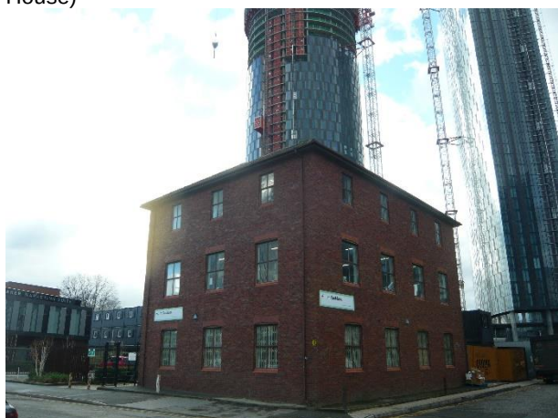
Photo 9: North-eastern and north-western elevations of Building 1 (Gaddum House)
