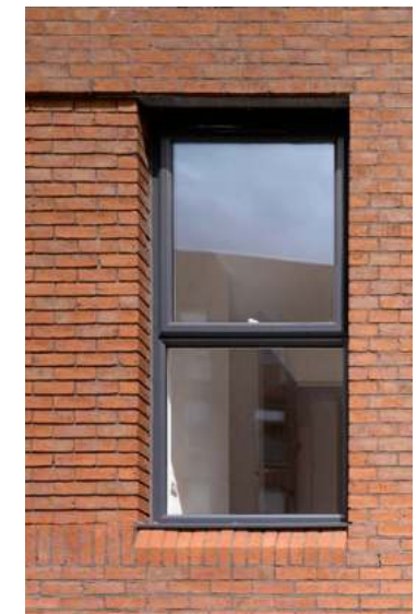
RAKED MORTAR JOINT PRECEDENT
