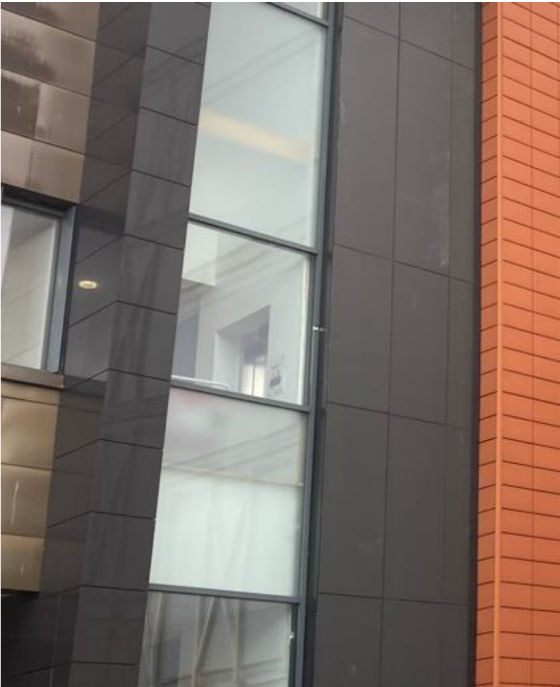
Existing entrance cladding in situ to the right of Oak Road Entrance (Joseph Holt Entrance) elevation.
