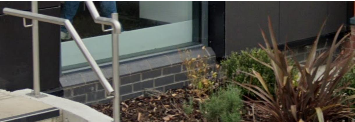
Existing brick plinth along Joseph Holt Entrance elevation to the left of the site.
