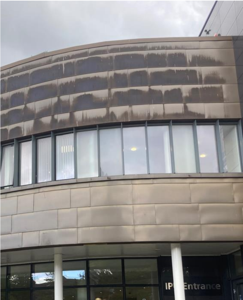
Existing brass claddings which wraps around the Oak Road Entrance elevation to the left of the site.
