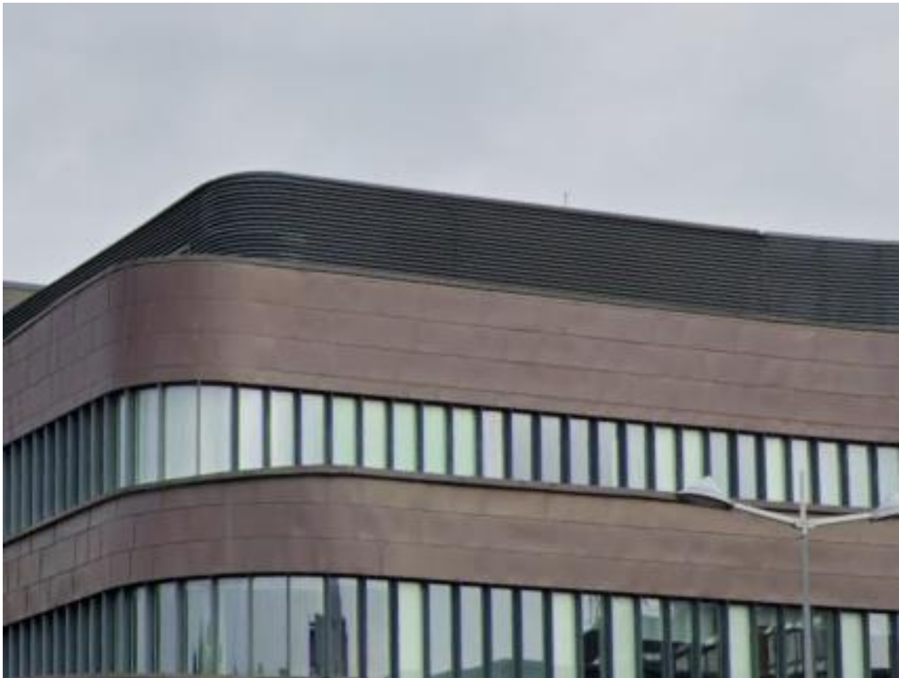
Existing louvred screening which runs around the top level of the Oak Road Treatment Centre.
