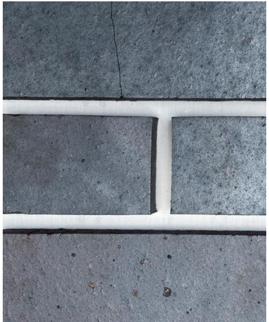
4 Oak Road Brick Plinth
