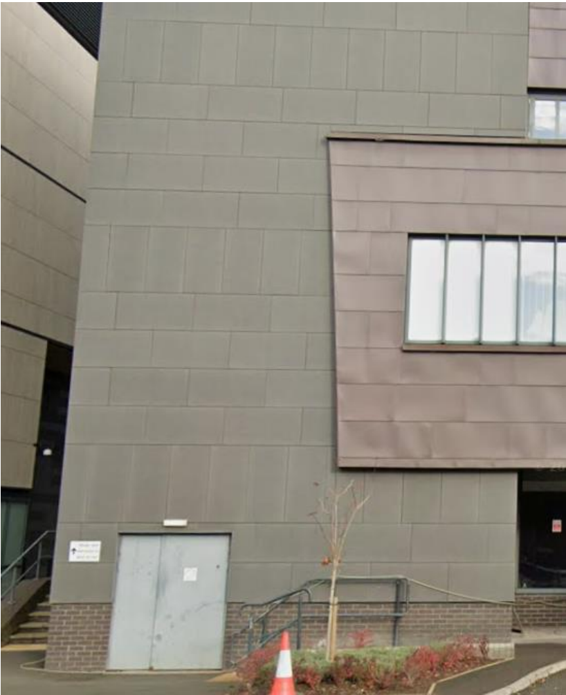
Existing 'bookend' cladding in situ at end of Oak Road Treatment Centre elevation.
