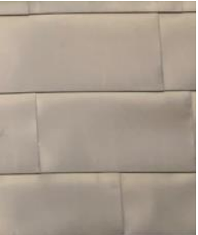
3 Oak Road Feature Cladding: Brass rainscreen
