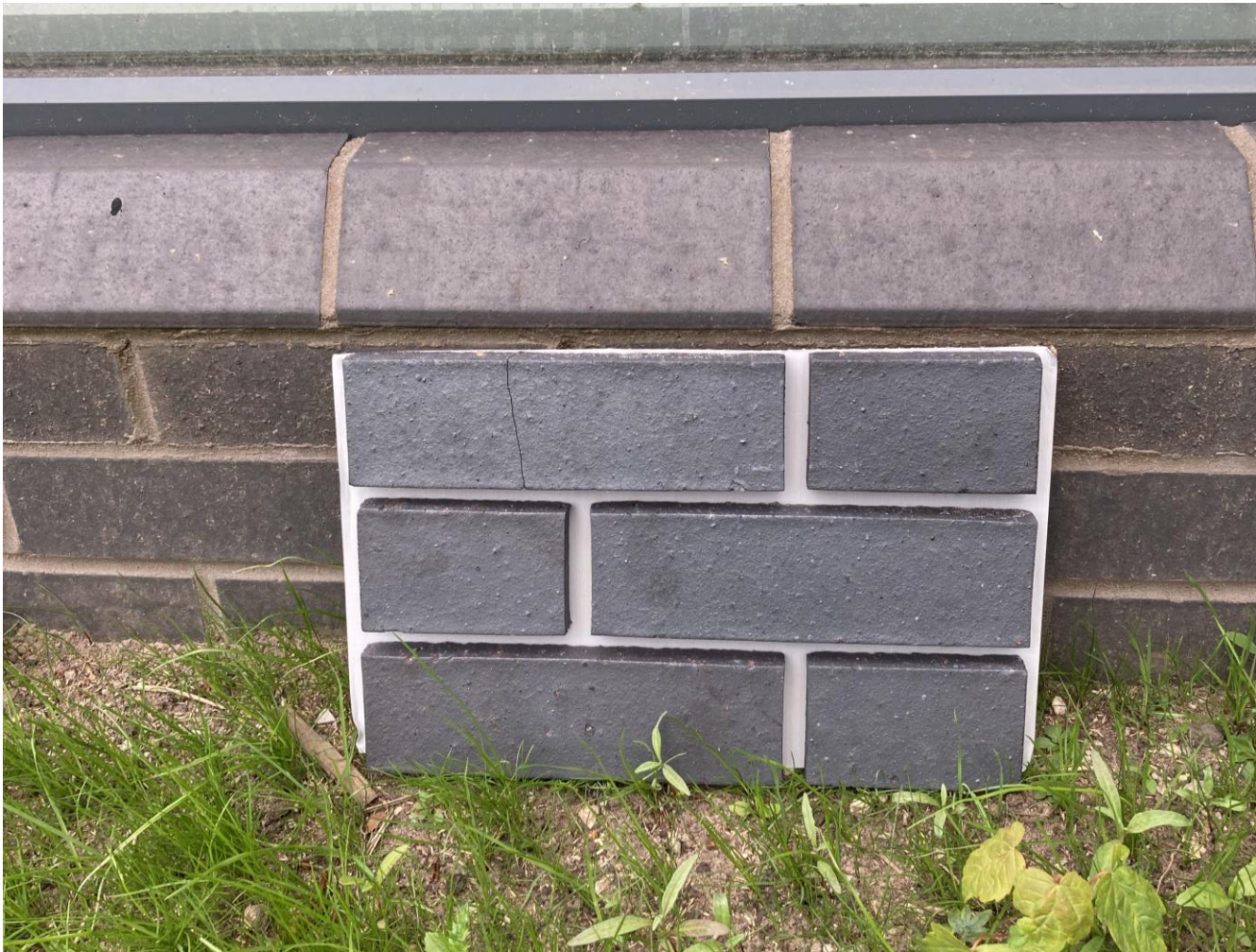
Lancashire Brick Lancrete Blue sample panel against Joseph Holt brick plinth (photograph taken on site)
