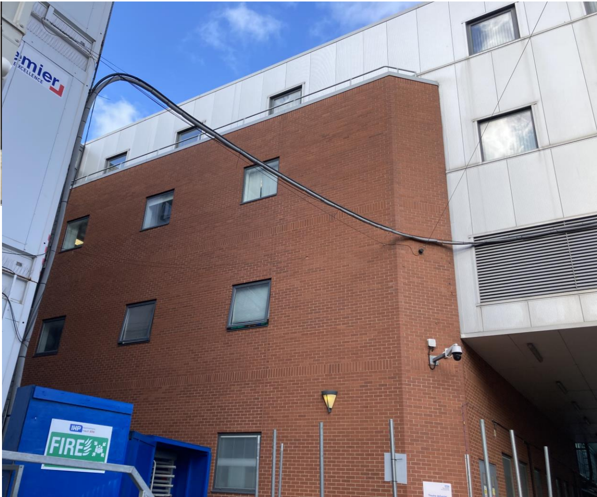
Existing facing brick to Block 34.
