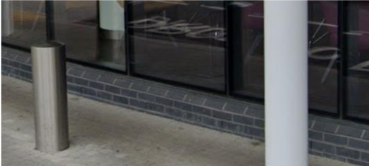
Existing brick plinth around the Oak Road Entrance elevation to the left of the site.
