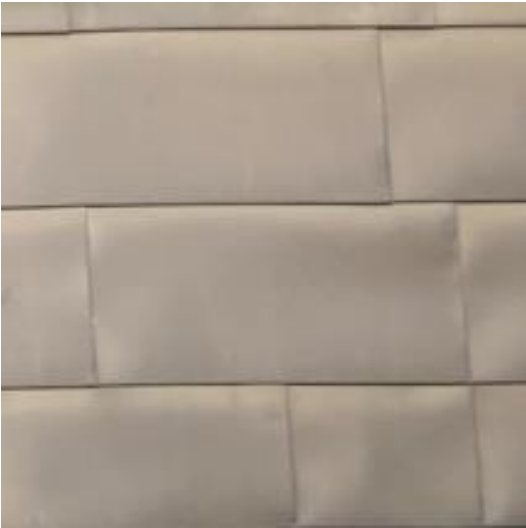
TECU Brass 70/30 Alloy photograph taken of cladding on site
