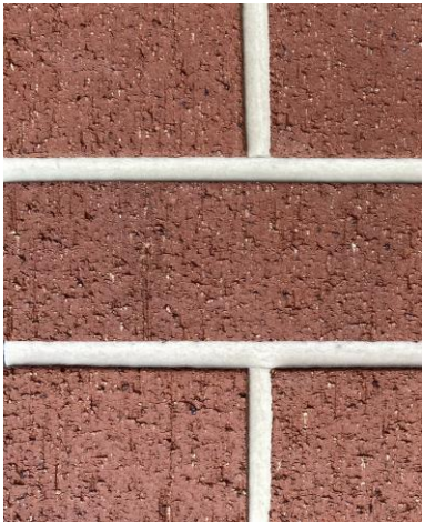
5 Block 34 Brick Infill
