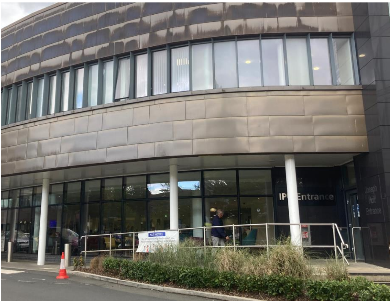
Existing curtain wall which runs around the Oak Road Entrance at Ground Floor.
