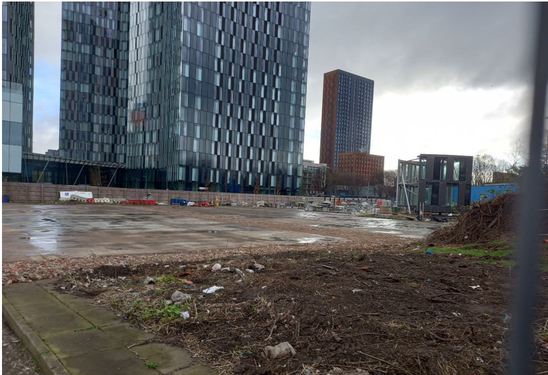
Photo 3: Facing south-east, showing eastern half of the site formerly occupied by commercial units which are now demolished. Storage of materials including traffic management, spare building equipment along the eastern and south-eastern site boundary.
