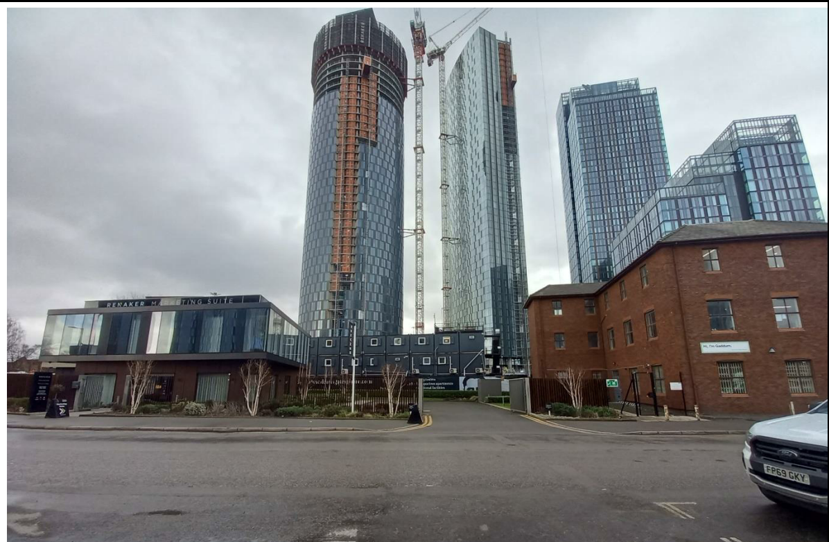
Photo 1: Facing west, showing western half of the site with semi-temporary marketing suite building (left), commercial building (No. 6 Great Jackson Street) and storage containers (back).
