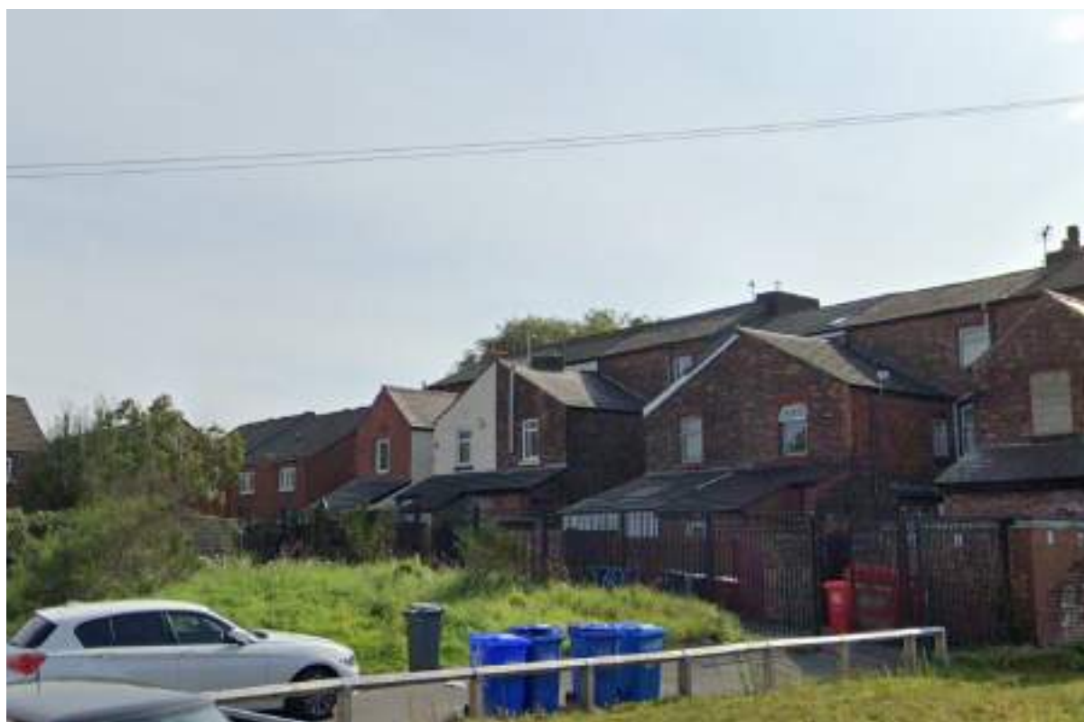
Photograph 1 – Site area at the rear of the residential properties
